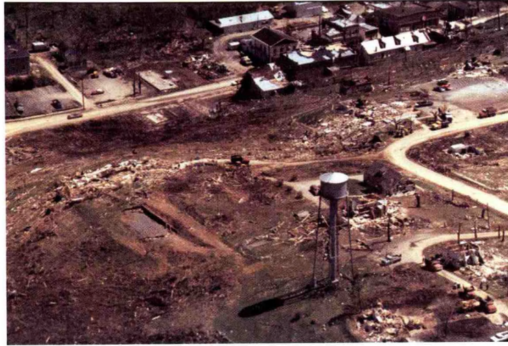
Figure 26. A water tower still standing near homes with no standing interior walls (Photograph courtesy of J.H. Golden, used by permission).
