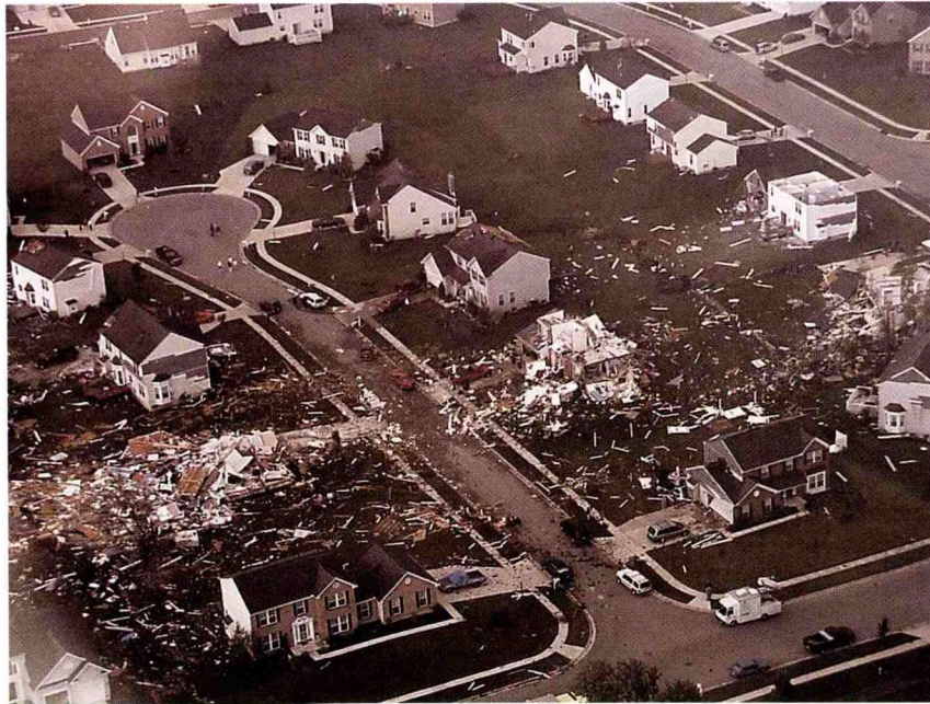
Figure 11. Path of a tornado in Xenia, OH, on 20 September 2000, showing near total destruction of one home (lower left) even as nearby homes have suffered virtually no structural damage. This is unlikely to be the result of extreme winds but is more likely to be a structural failure associated with that particular home, and is complicated by the damage to the home across the street, which surely produced many projectiles. (Photograph courtesy of J.H. Golden, used by permission).
