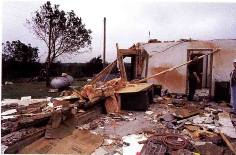
Figure 29. Damage to a poorly constructed garage implies much stronger winds than the nearby tree, which has one broken tree branch but is otherwise not heavily damaged (FEMA photograph by C. Doswell).
