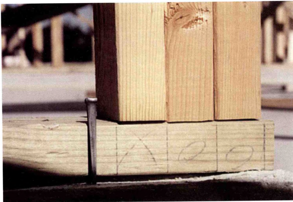
Figure A2.4. Cut nail, often powder-driven, used to attach bottom plate to foundation slab after the concrete has hardened. Note the relatively shallow penetration of the cut nail. Often, the impact of the nail shatters the concrete, leaving the nail essentially unattached to the concrete beneath the bottom plate. [Photograph © T. Marshall, used by permission]
