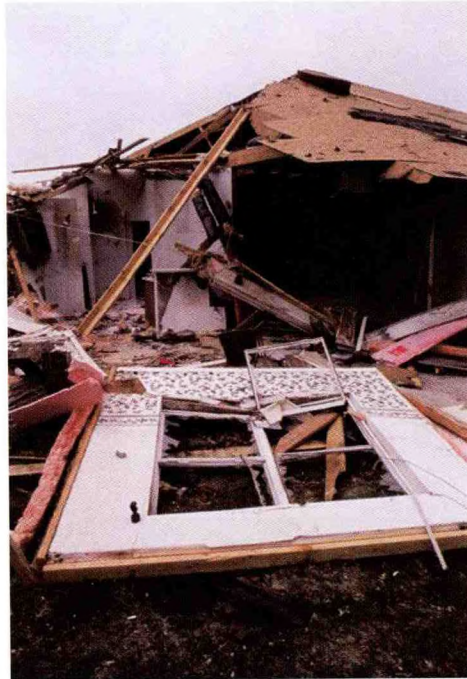
Figure 43. (Previous page) A frame home with little or no damage on its front , the side of the home facing the tornado. Note the damage to the home behind that in front, farther from the tornado (which has lost much of its roof), and the debris filling the space between homes in front. (Above) Damage to the rear of the home seen in the top photograph, caused by elements of the roof from the home across the street, behind it (FEMA photographs by C. Doswell).
