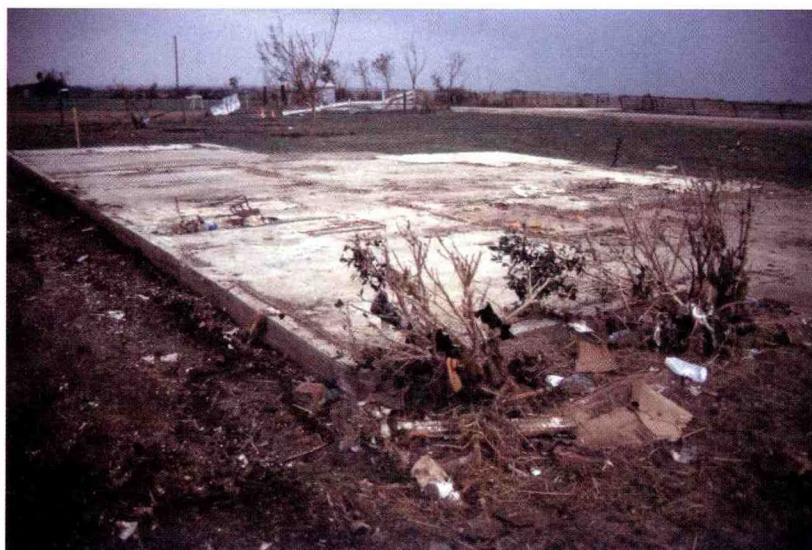
Figure 27. Empty slab left in the Double Creek Estates subdivision following the tornado of 27 May 1997 in Jarrell, Texas (Photograph © courtesy of T. Marshall, used by permission).
