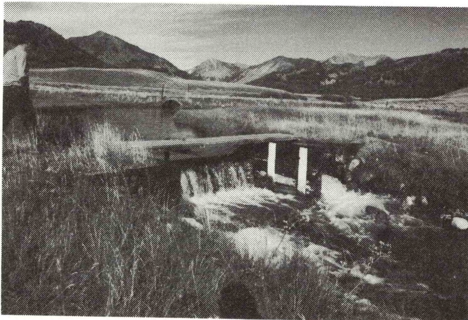
FIGURE 7. - WOOD AND CONCRETE WING DAM USED TO DIVERT WATER INTO IRRIGATION DIVERSIONS. THESE STRUCTURES ARE NOT AS ABUNDANT AS THOSE FOUND IN FIGURE 6.
