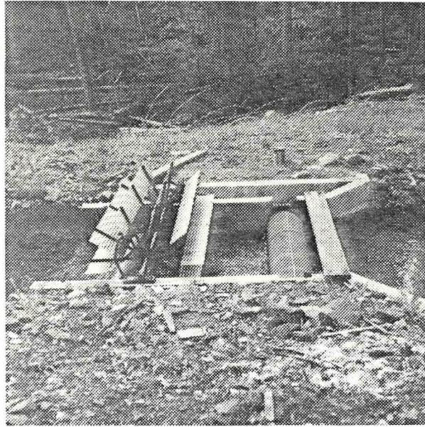
Figure 9 - A paddle wheel operated drum fish screen in operation on a tributary of the Salmon River in Idaho. Water flow is from right to left.
