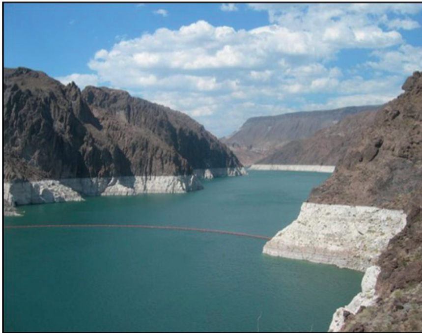
FIG. 1. Low water levels at Lake Mead (Nevada), shown as white bathtub rings and highlighting the importance of quantifying reservoir evaporation (credit: Kyle Simourd, CC 21). Between the high water mark in 1942 (33,000,000,000 m 3 ) and the present photo (2015), the lake has lost about 66% (21,000,000,000 m 3 ) of its water, based on stage and storage data at Hoover Dam ( http://goo.gl/flktcft ). According to the U.S. Bureau of Reclamation, Lake Mead's water level reached an all-time low in May 2016 (Jacobo 2016).
