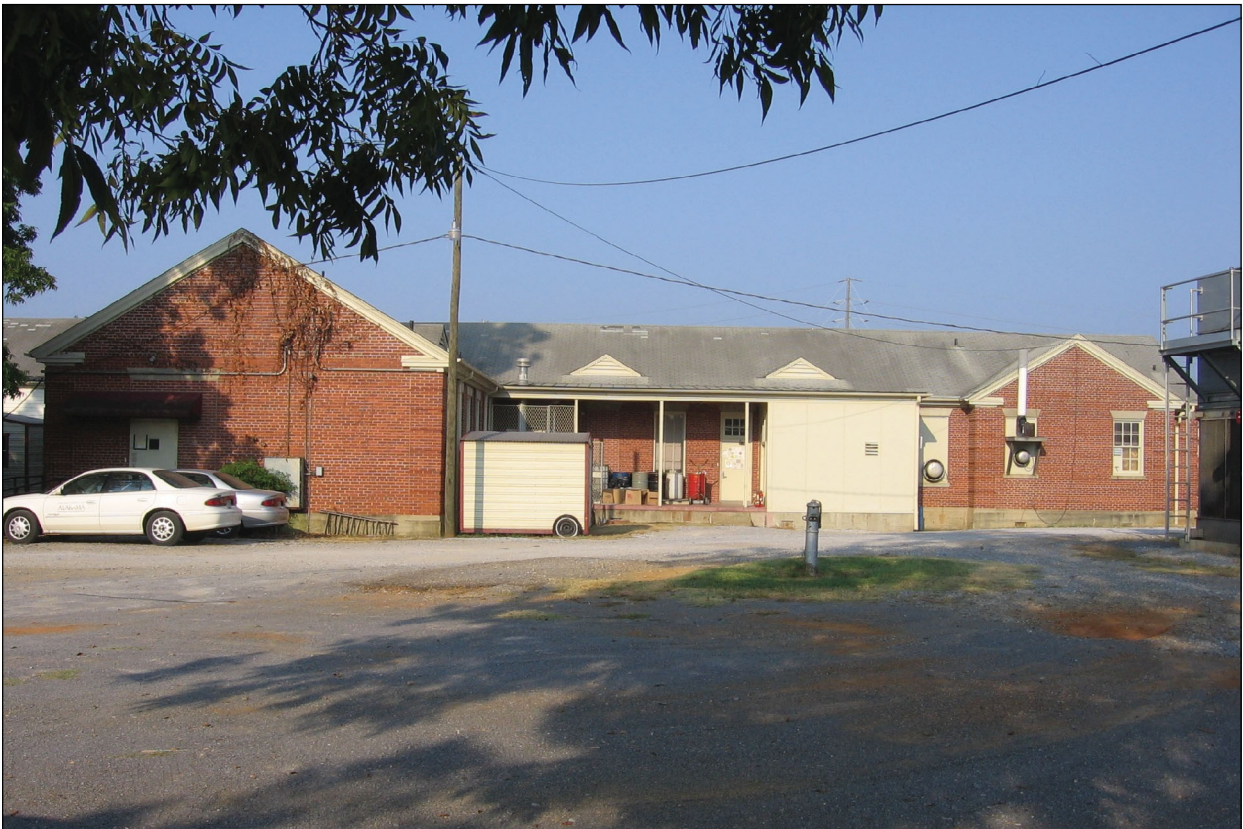
Figure 3-D. Rear (eastern) façade of existing Environmental Health and Safety Building. Date taken: 9/21/2010
