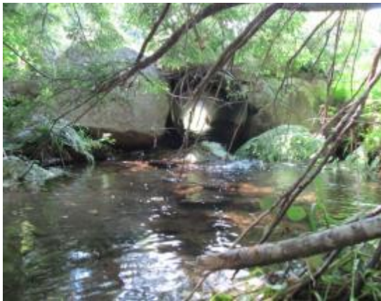
Figure 5.7.3. Above left photo shows the culvert inlet prior to replacement. The above right photo shows the post construction waste block bridge. The three foot culvert was replaced with a 14 foot bridge.
