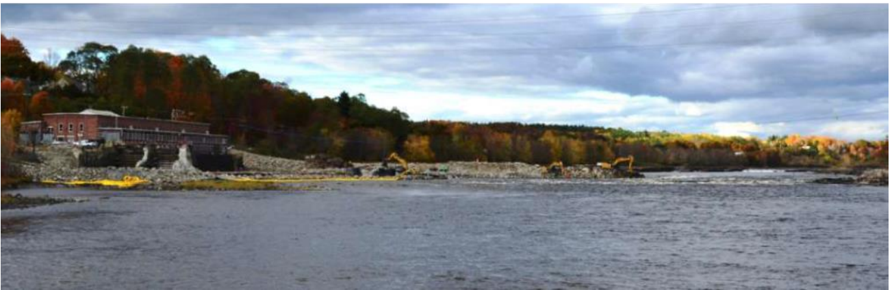
Figure 5.4.1 Aerial view of the Veazie Dam on the Penobscot River before removal (top photo) and the view near the end of destruction in September 2013.
