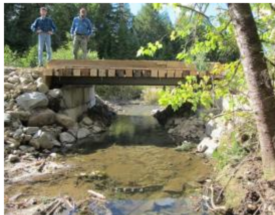
Figure 5.7.3. Above left photo shows the culvert inlet prior to replacement. The above right photo shows the post construction waste block bridge. The three foot culvert was replaced with a 14 foot bridge.
