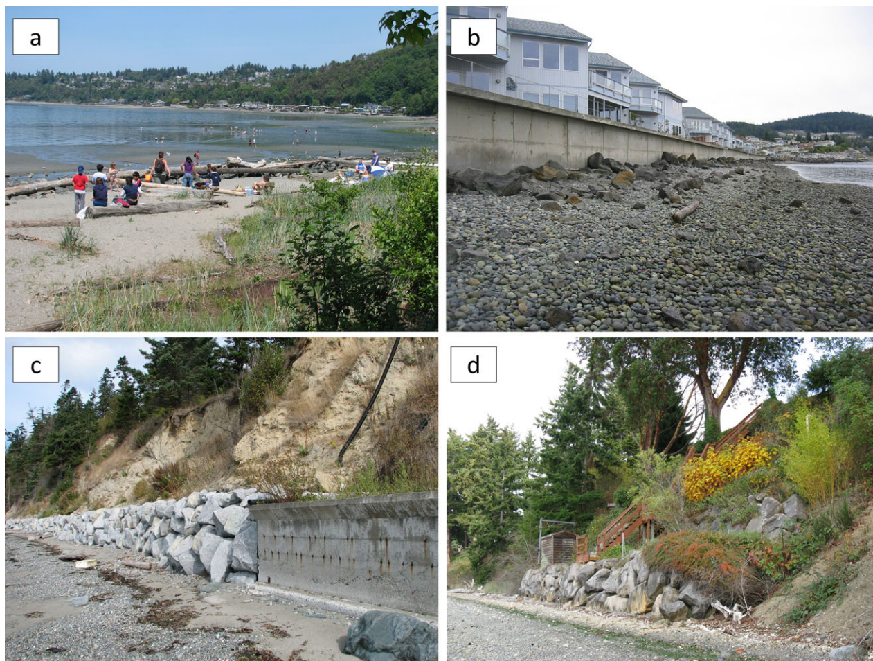
Figure 1 Examples of EFGS or their losses on beaches in Puget Sound. (a) Recreational enjoyment in a natural area of Seahurst Park; (b) condominiums built on fill retained by a low-elevation concrete bulkhead; such armoring impacts EFGS by all four mechanisms in Table 1; (c) former feeder bluff with sediment impounded by armoring; and (d) stairs to the beach protected by a rock bulkhead. All photos by Hugh Shipman.
