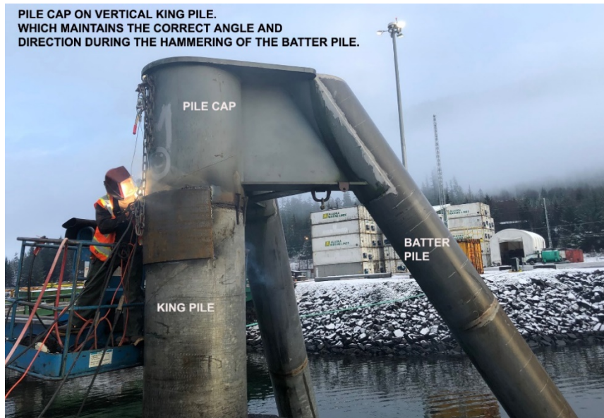
FIGURE 3: Vertical and Diagonal Piles with Pile Cap
