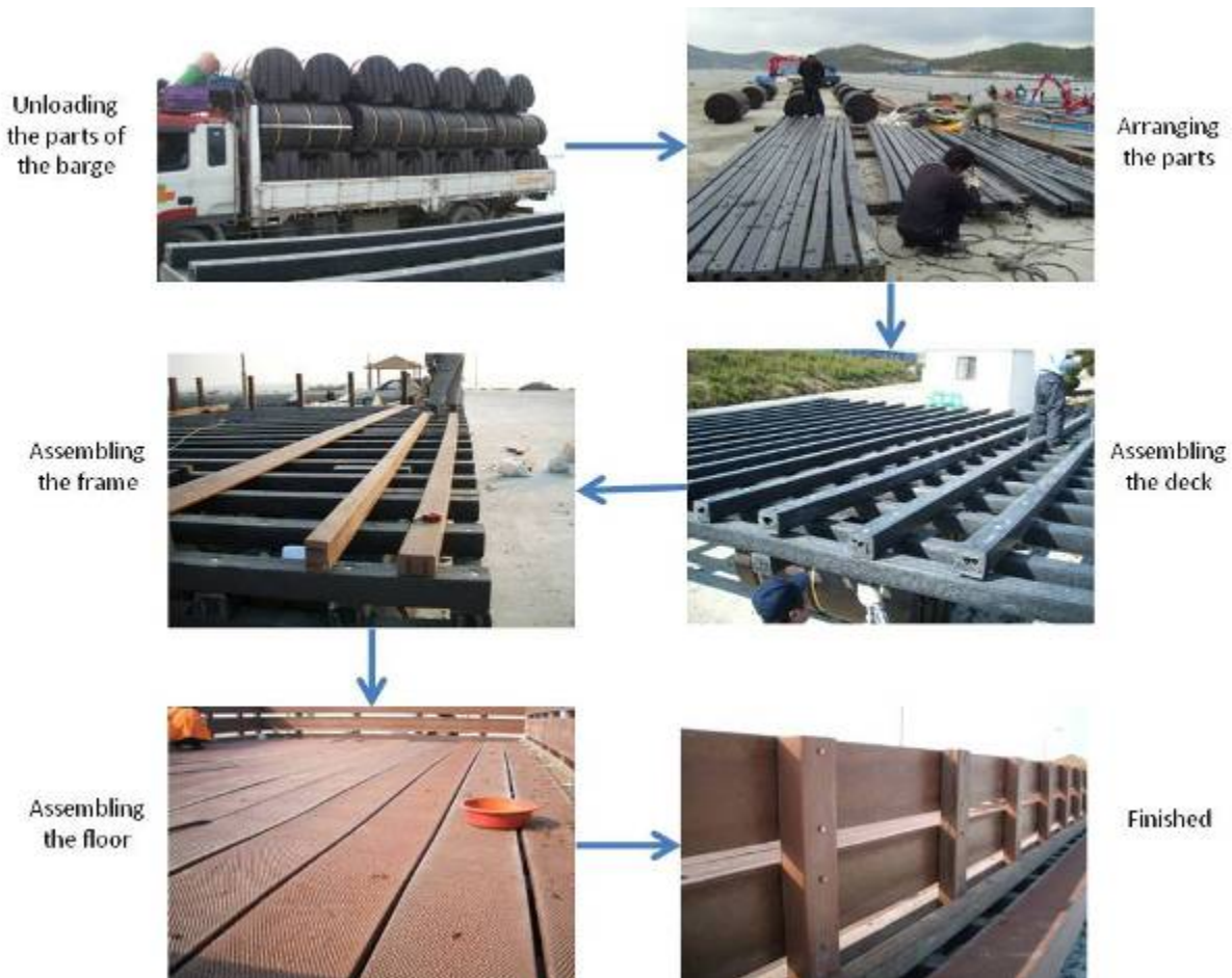
Figure 1. Process of building a floating receptacle for marine litter.
