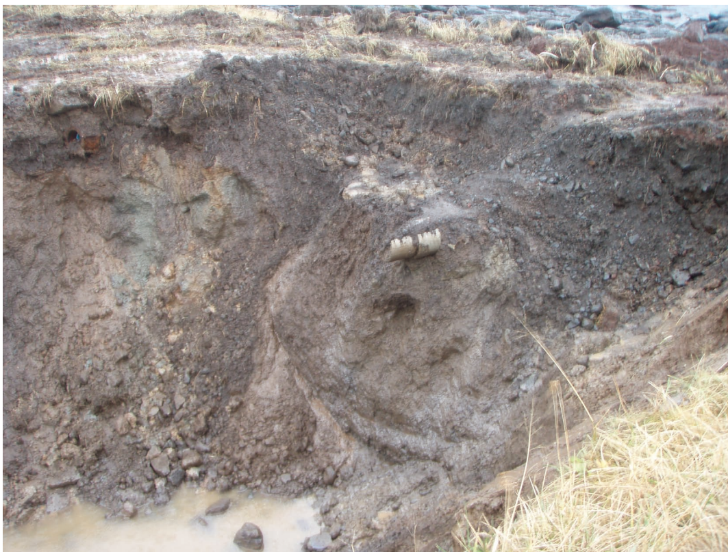
Photograph 10. NOAA Site 29 East Excavation 23 October 2006 View of asbestos-cement pipe left behind in Bering Sea buffer set-back. Note beach in upper right. Looking northwest.
