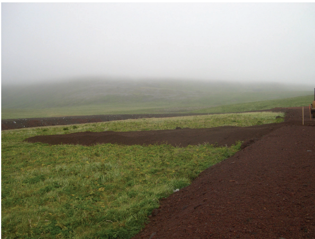
Photograph 13. New City Landfill 9 September 2006 View of ramp built into interior of the City of St. George's new landfill site to allow access for stockpiling petroleum-contaminated soil for use as municipal waste day cover. Looking east.
