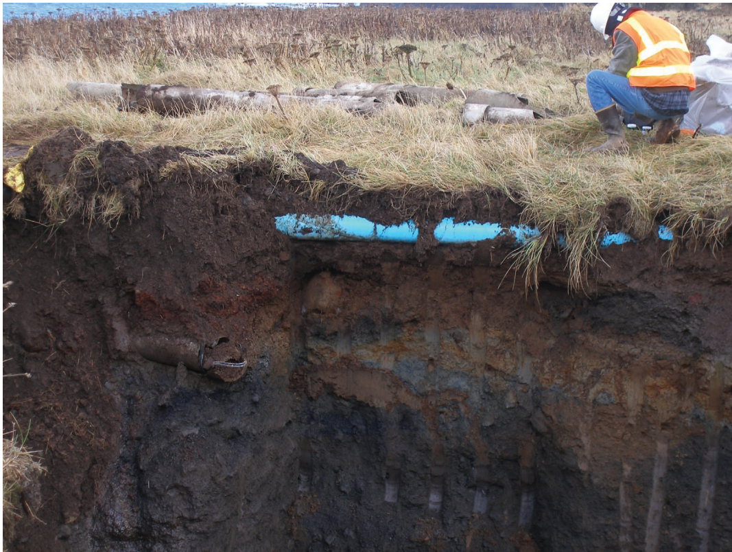
Photograph 7. NOAA Site 29 East Excavation 20 October 2006 View of abandoned blue plastic discharge line from the inactive fish processing plant which crossed over the abandoned asbestos-cement sewer line (in photo center left). Looking northeast.
