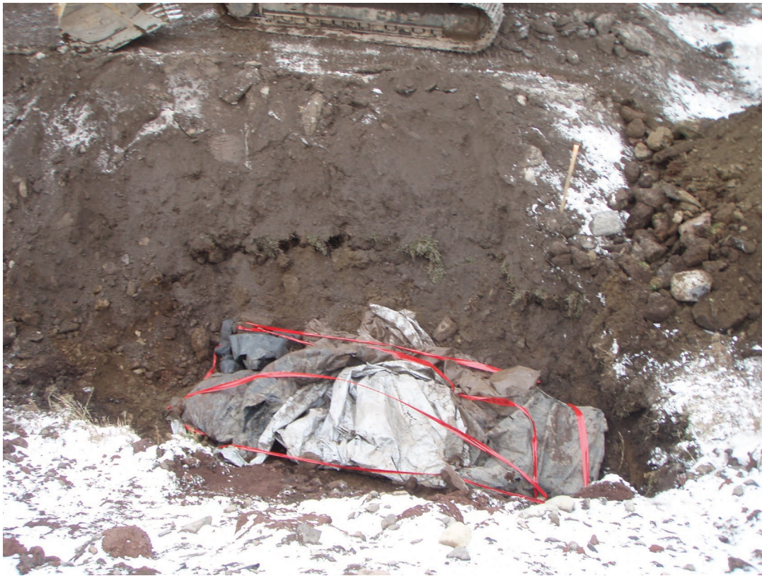
Photograph 15. New City Landfill 11 November 2006 Asbestos-cement pipe, covered with liner and asbestos caution tape, prior to burial at the City's new landfill.
