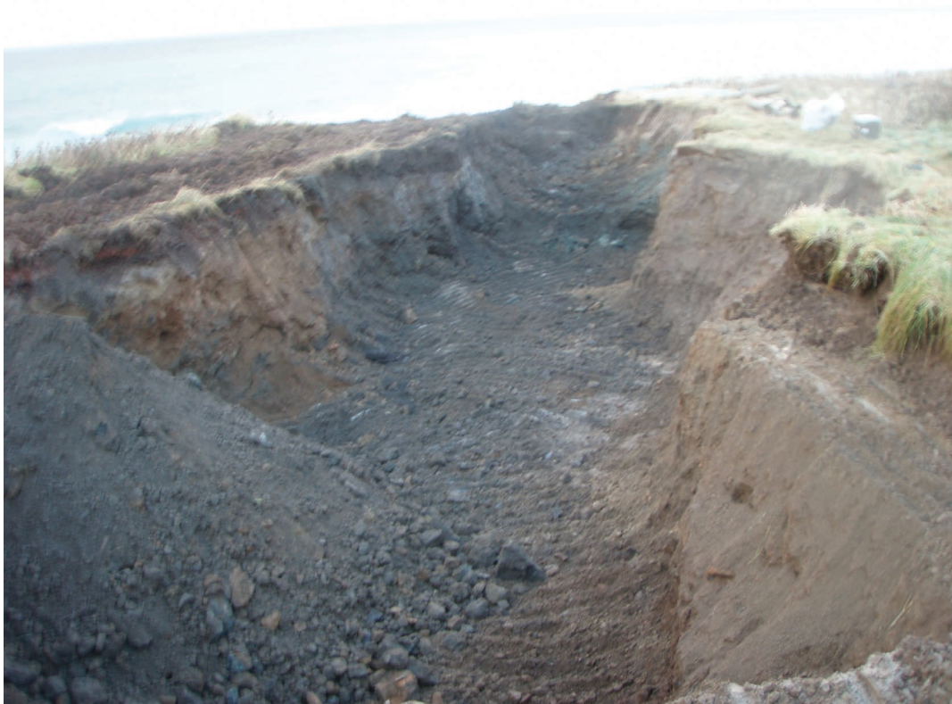
Photograph 8. NOAA Site 29 East Excavation 20 October 2006 View of contaminated soil excavation that followed an abandoned asbestos-cement pipeline. Looking northeast.
