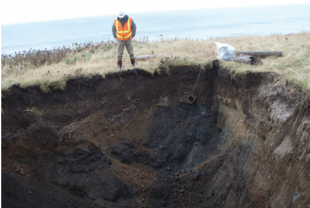
Photograph 6. NOAA Site 29 East Excavation 18 October 2006 View of grey soil that was contaminated by both sewage leakage from the asbestos-cement pipe and fuel from leaking aboveground pipelines that traveled sub-surface along the asbestos-cement pipe. Steven McCain, ChemTrack Project Manager, in photo. Looking north-northeast.
