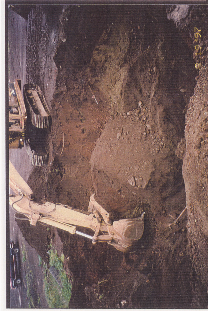
Figure 3. TPA 22-5, The Gas Station #1 UST, Excavating Contaminated Soil.
