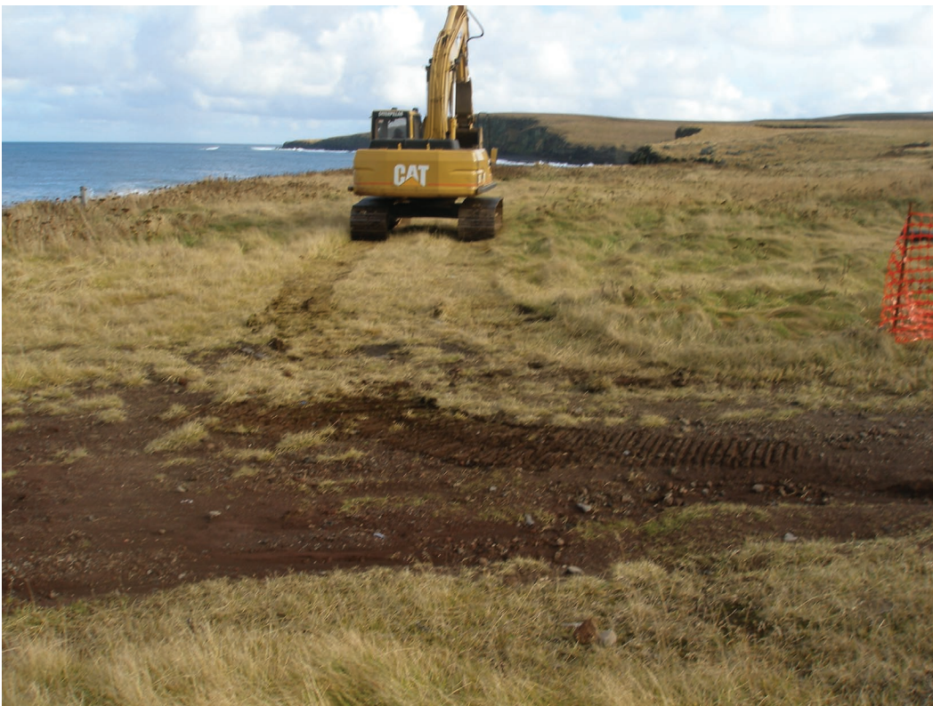
Photograph 2. NOAA Site 29 East Excavation 18 October 2006 View of NOAA's Caterpillar 320B excavator moving onto the site. An old road bed was found beneath the tundra grass, allowing access without the need for building a temporary road. Looking northeast.
