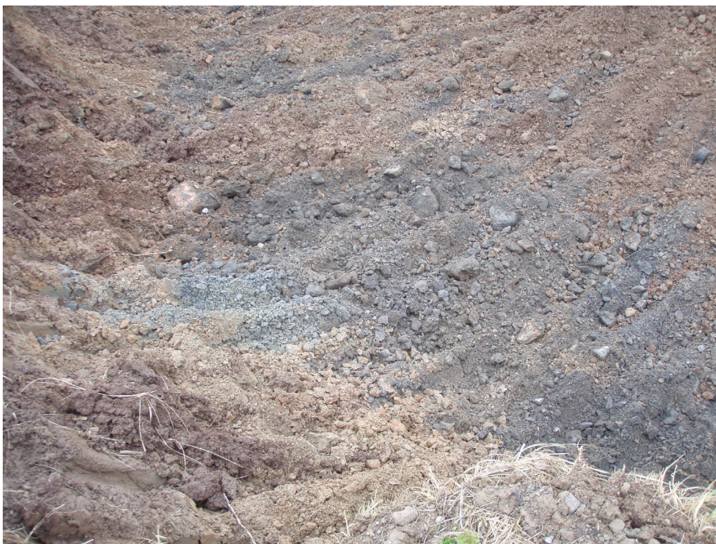
Photograph 21. NOAA Site 29 East Excavation 11 May 2007 Grey diesel-range organics (DRO) contaminated soil.
