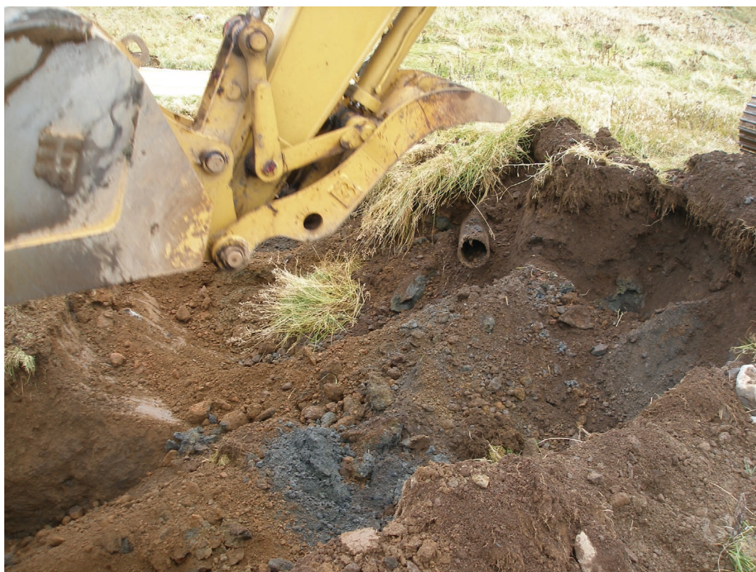
Photograph 4. NOAA Site 29 East Excavation 18 October 2006 View of grey petroleum-contaminated soil layer and an abandoned 8-inch diameter asbestos-cement pipe encountered at about three feet below the ground surface. Facing southwest.
