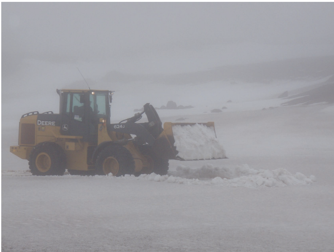
Photograph 16. Scoria Borrow Pit 9 May 2007 Clearing snow at scoria backfill borrow area to enhance melt and ground thaw.
