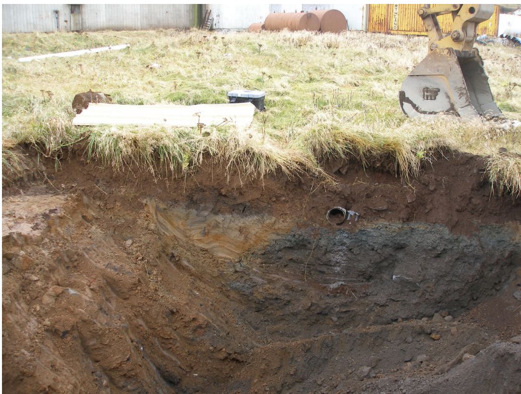
Photograph 5. NOAA Site 29 East Excavation 18 October 2006 Grey contaminated soil layer and asbestos-cement pipe exposed during the excavation. Looking southwest.
