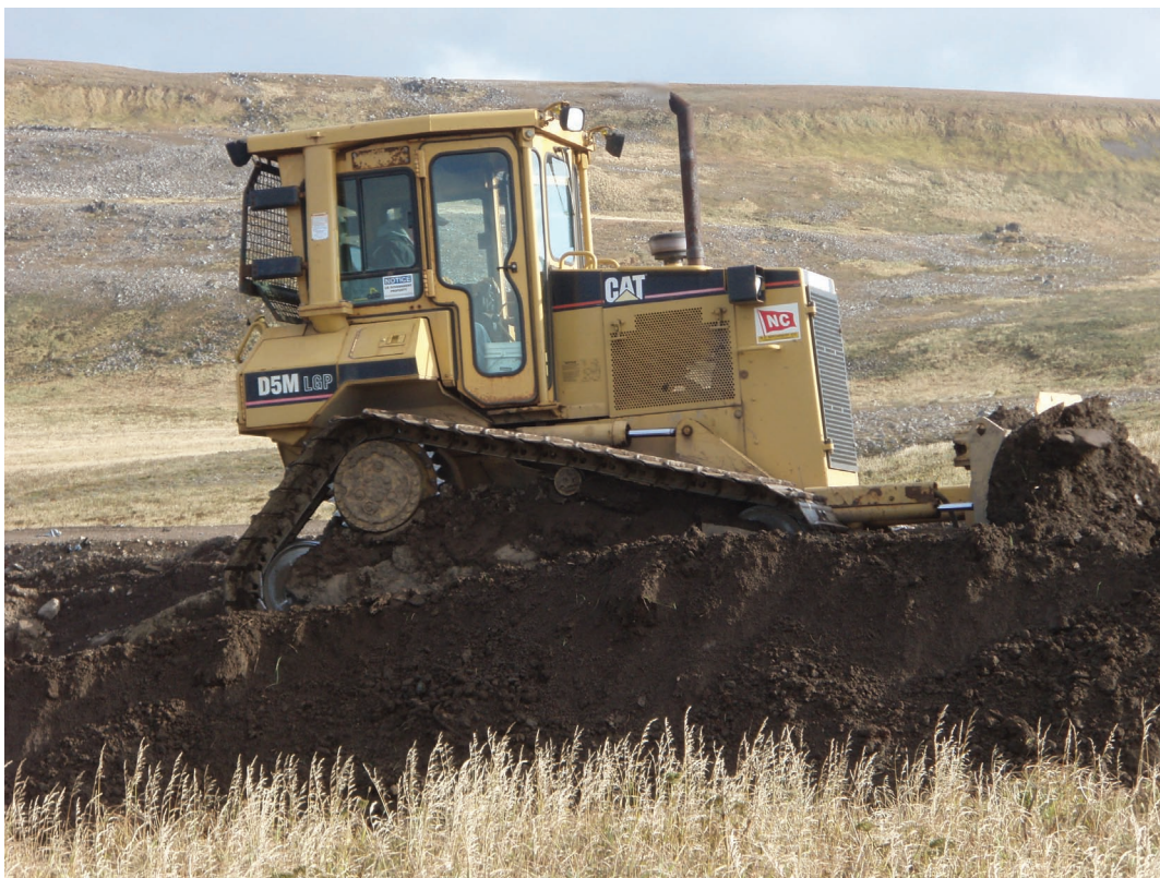
Photograph 14. New City Landfill 7 October 2006 Pushing soil into five foot high municipal waste day cover stockpiles at the new landfill. Looking northeast.
