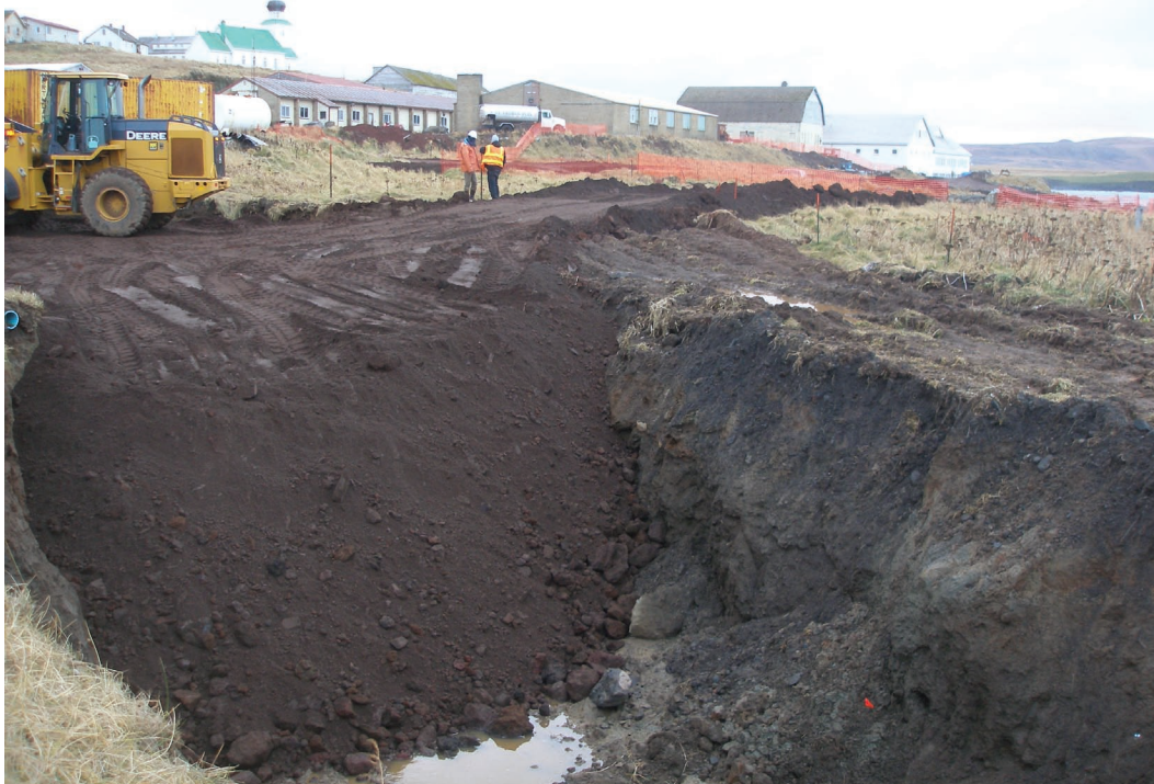
Photograph 11. NOAA Site 29 East Excavation 3 November 2006 Backfilling excavation around Hart Crowser sample location EO-SS-3; see Figure 6 of the report. Looking southwest.
