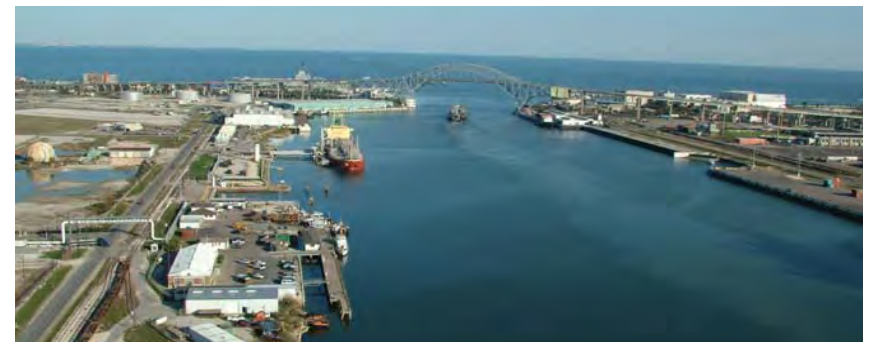
Port of Corpus Christi, TX. Credit: Port of Corpus Christi Authority
