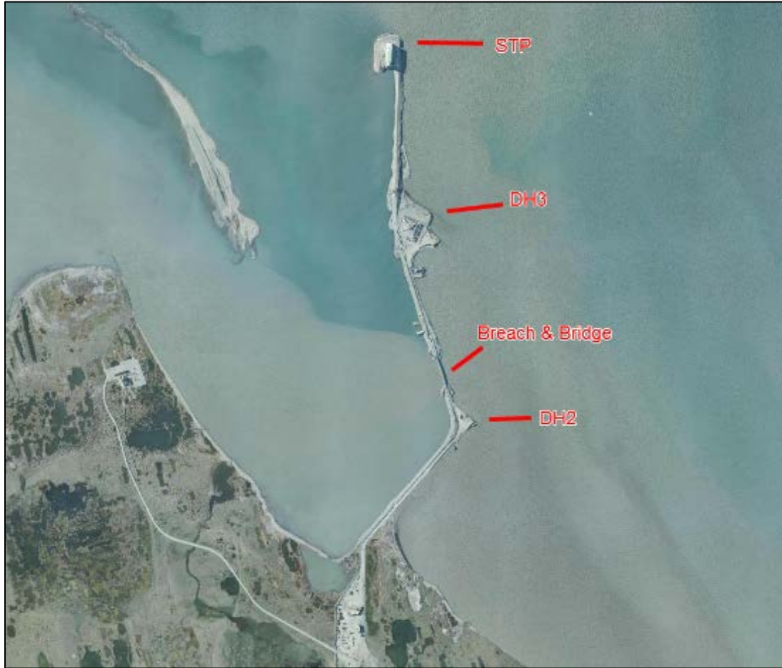
Figure 2. Existing conditions at West Dock in Prudhoe Bay, Alaska
