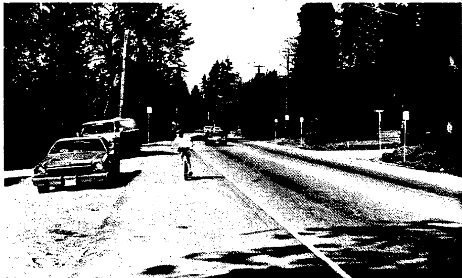
SR 527 looking north. The proposed sidewalk will extend approximately from the pavement edge to the cyclist.
