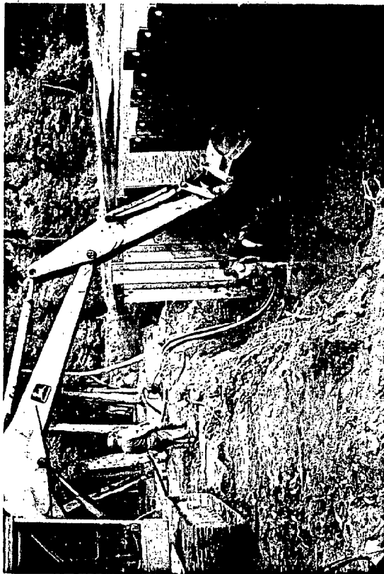
17. Temporary cofferdam constructed by N. H. Rabell and Sons, Inc. prior to construction of the new boat ramp.
