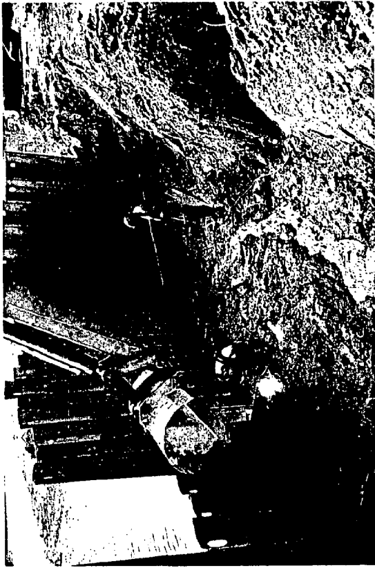
18. Construction workers weld the base of the cofferdam. July/Aug. 1988
