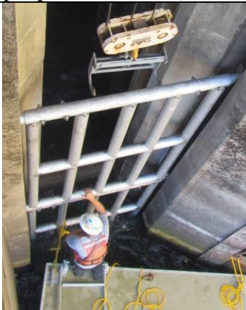
New LL1 SLED being installed (10/4/2017)
