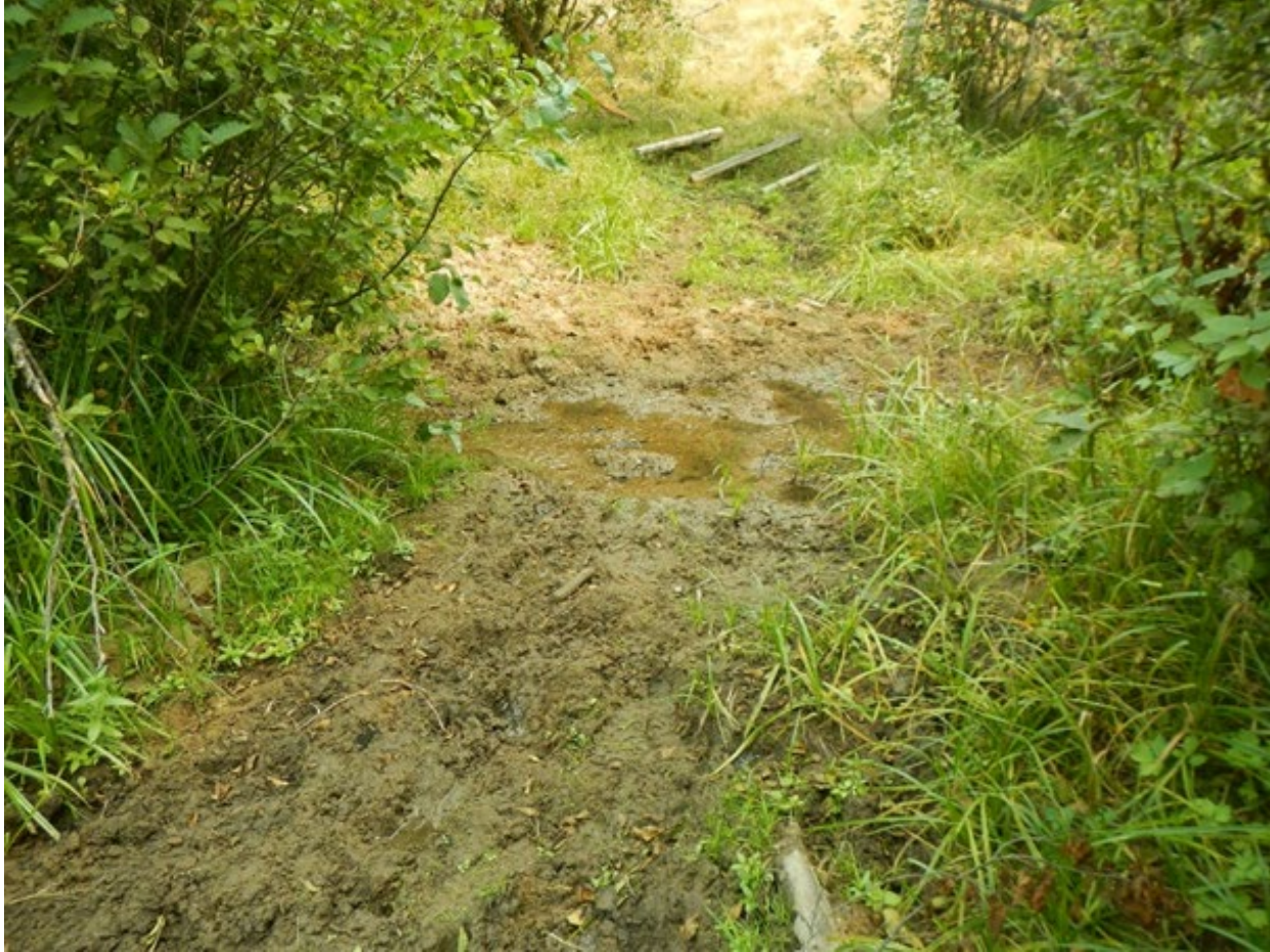
Figure 4: Road 820313, unimproved ford of unnamed tributary to Ruby Creek
