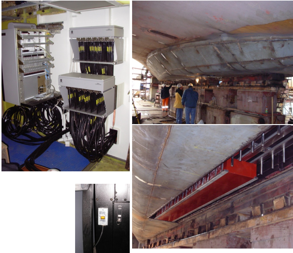
Figure 3. Photos: (Clockwise from left) EM 302 TRU unit, Transducer fairing, Elements of EM 302 being installed inside the fairing, TRU remote on / off switch.
