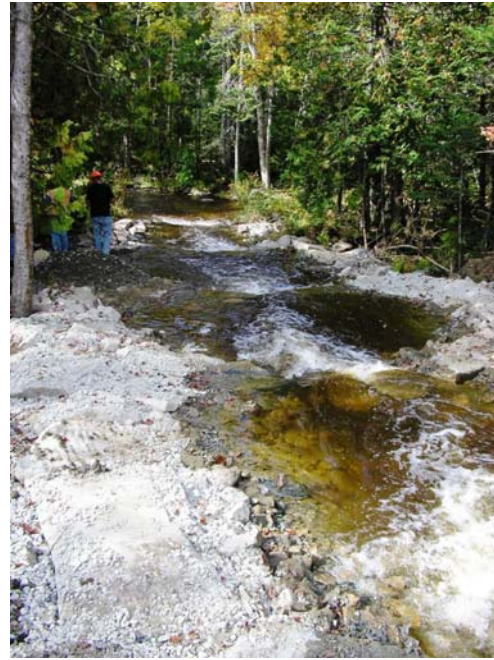
Figure 5.7.3 Before and after photos of Flanders Stream, Sullivan, ME. Photo on left shows Denil fishway and culvert combination. Photo on right shows functioning rock/weir pool.
