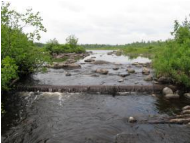
Figure 5.7.5 Roaring Brook - The above remnant log drive dam on Roaring Brook in the Pleasant River drainage was identified in late June of this year by NRCS's Fisheries Biologist. The dam held back over a half mile of dead water habitat creating a thermal barrier for cold water fish species like brook trout and Atlantic salmon. The removal of the dam has reduced the half mile impoundment above the dam site and has connected an additional seven miles of stream. NRCS provided the coordination, land owner contacts and technical assistance for this project. Partners included Elliottsville Plantation Inc., USFWS, DMR, MDIFW and TU.
