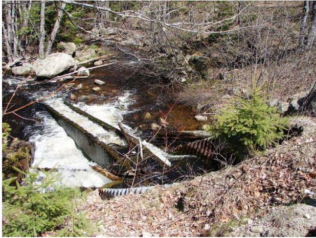
Figure 5.7.3 Before and after photos of Flanders Stream, Sullivan, ME. Photo on left shows Denil fishway and culvert combination. Photo on right shows functioning rock/weir pool.
