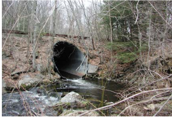
Measuring velocities inside Town Brook culvert. A downstream rock weir backfloods the outlet.
