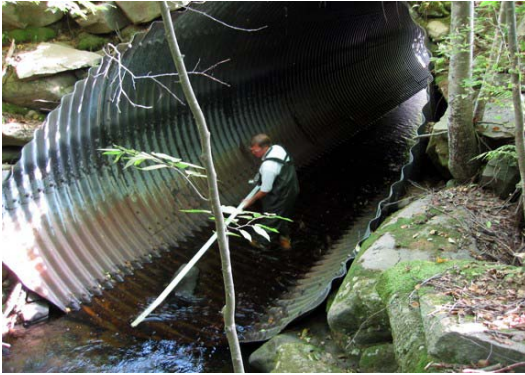
Measuring velocities inside Town Brook culvert. A downstream rock weir backfloods the outlet.
