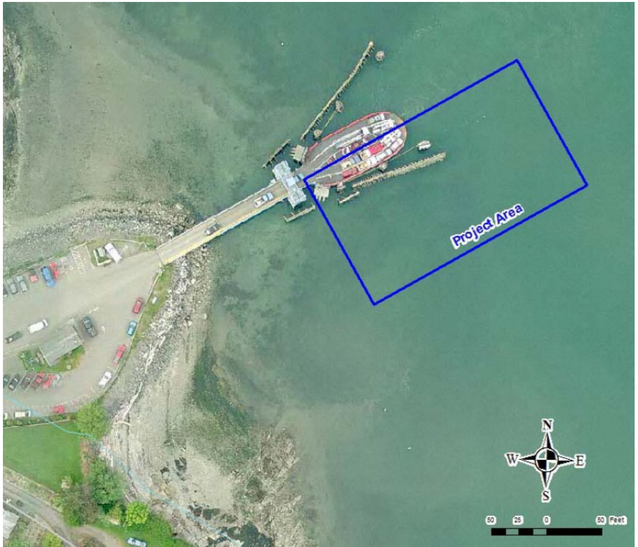
Figure 3. Aerial view of project area.
