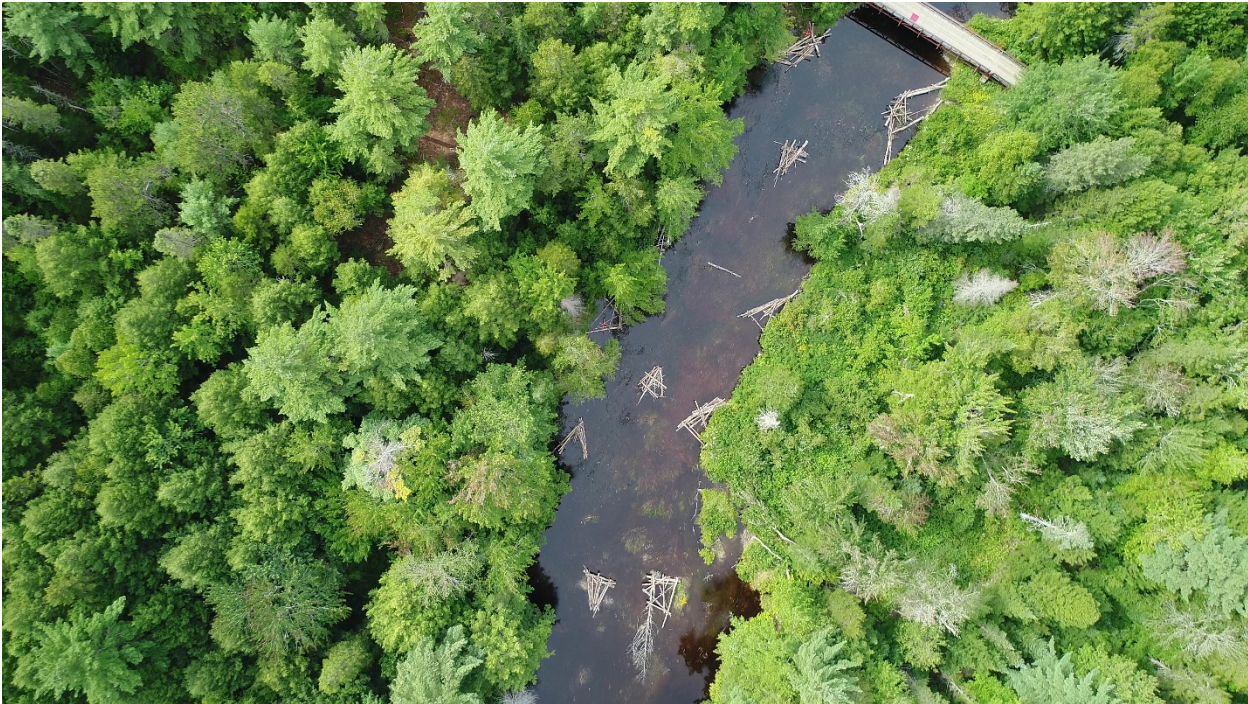
Figure 5.3.6 Aerial photo showing all 12 PALS constructed at the Ford Site, Narraguagus River, Maine, 2018. (photo credit: Chris Federico, Project SHARE)
