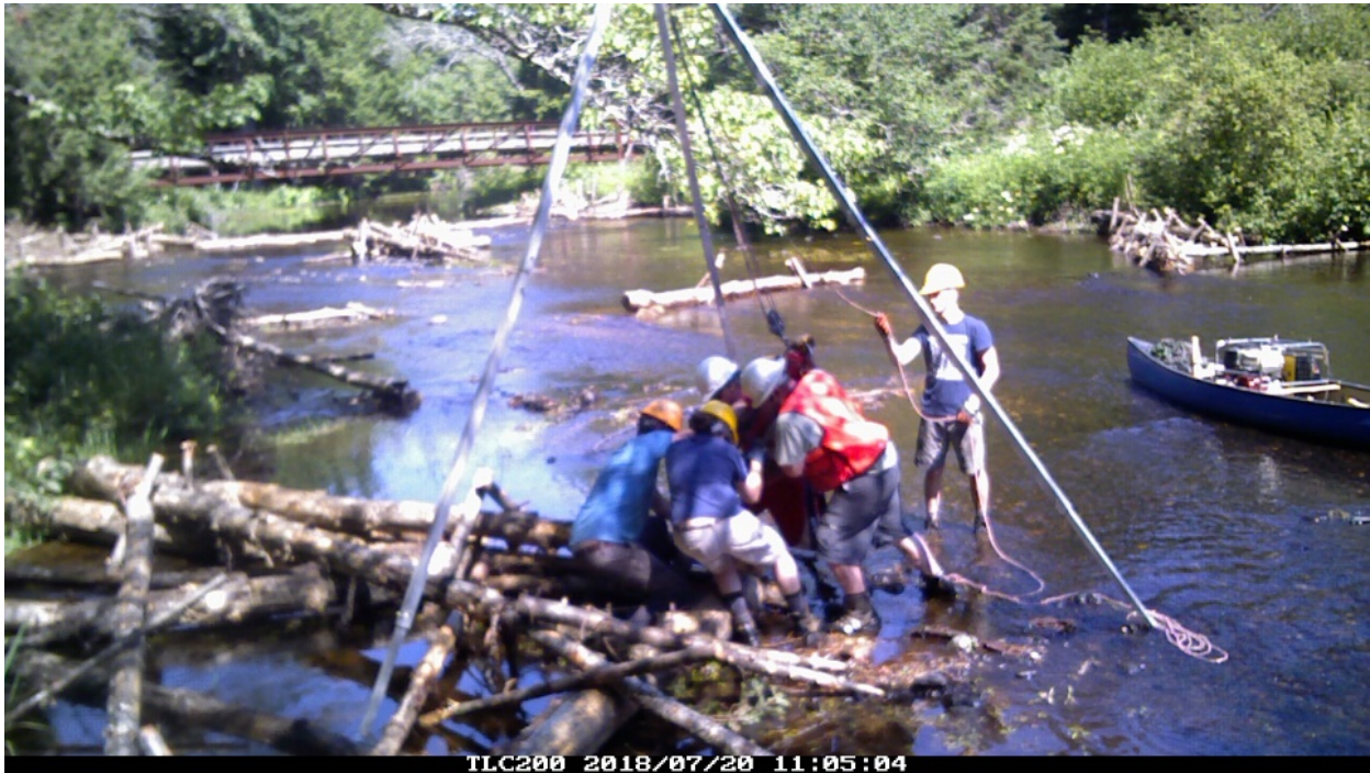
Figure 5.3.5 Driving a post into a PALS at the Ford Site, Narraguagus River, Maine, 2018. (photo credit: Chris Federico, Project SHARE)
