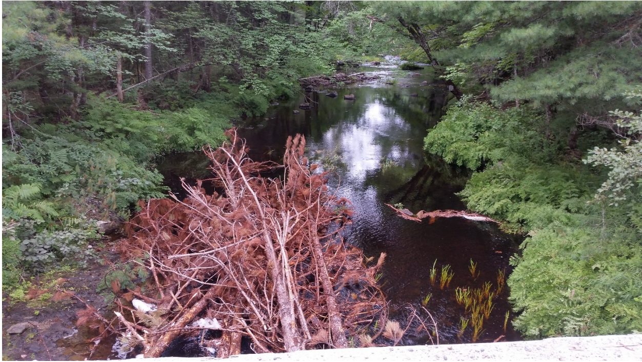
Figure 5.3.9 Commercially harvested red pine tree addition as self-placing wood, 31-00-0 Rd bridge, Narraguagus River, Maine, 2018. (photo credit: Chris Federico, Project SHARE)
