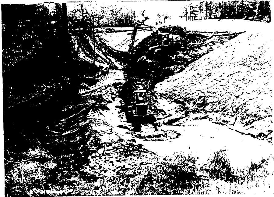
Figure E-1: A sediment trap being cleaned out. This is a very necessary task for traps which "silt-in".
