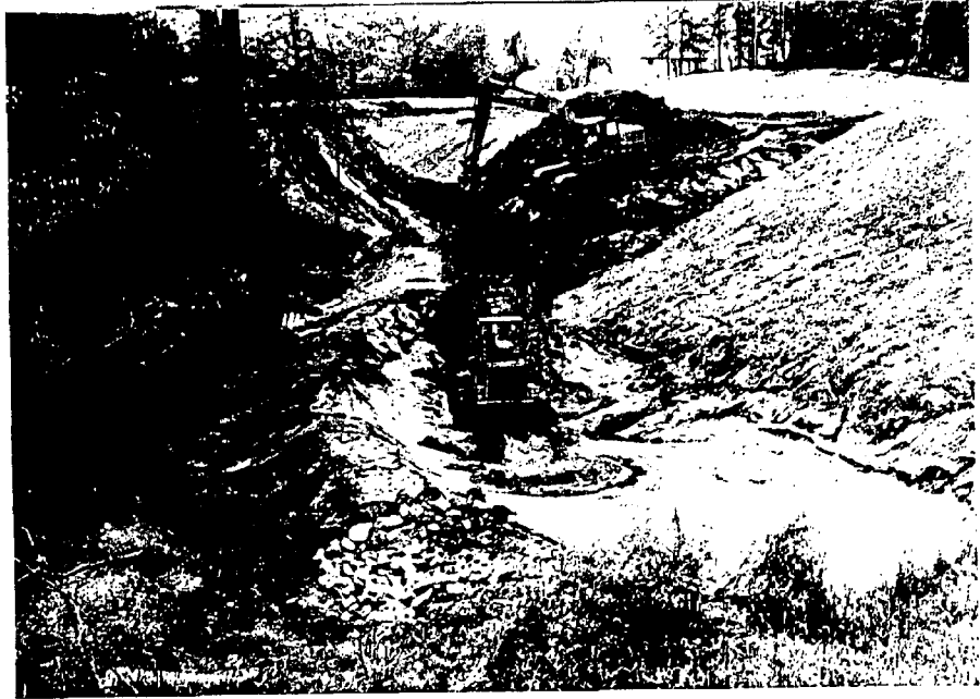
Figure E-1: A sediment trap being cleaned out. This is a very necessary task for traps which "silt-in".
