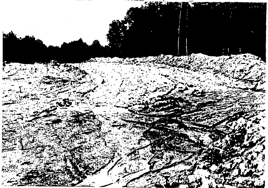
Figure D-6: With large disturbed areas draining to a single sediment trap, the NRD is sure to be polluted with large amounts of sediment.
