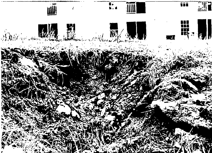
Figure D-3: Erosion and gullying usually start at the top of the slope, and this is where prevention should start.
