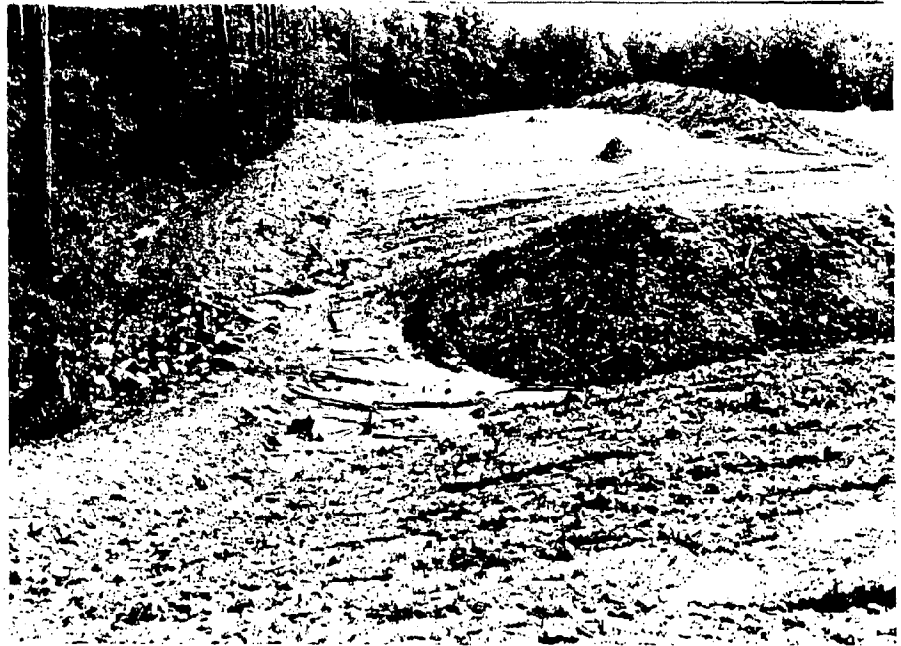
Figure D-5: This figure shows the large disturbed area which drains, along with all of its sediment, to the now filled in sediment pond. Such a situation will result in a large amount of sediment reaching the NRD.
