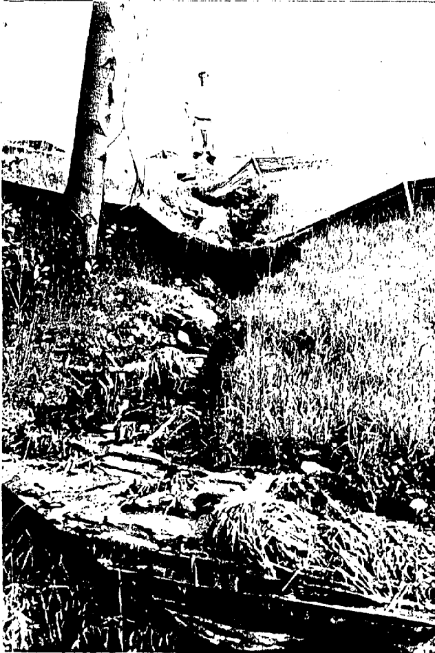
Figure A-4: This photograph is a view of the gulling and damaged silt fences looking up-slope from down near the stream.
