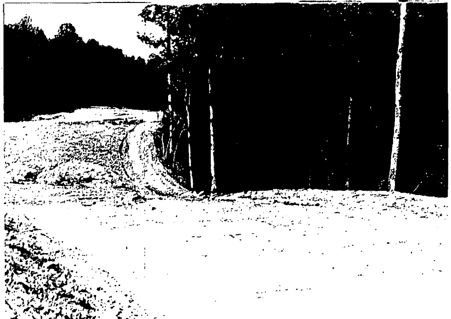
Figure E-2: Berms are a better barrier to stormwater and sediment than silt fences. The berm along the tree line here (also see Figures 3, 4, and 5) will prevent sediment from flowing down the slope and into NRD areas.
