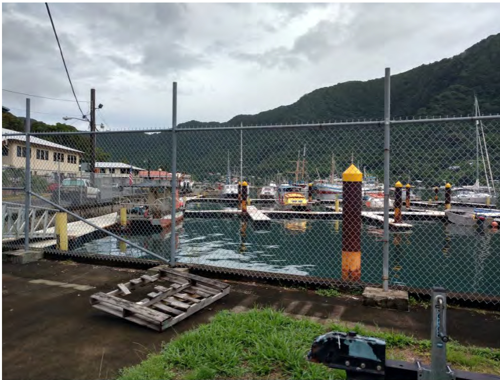
Figure 3. Setting of the proposed ice house at the DMWR site, inner Pago Pago Harbor.
