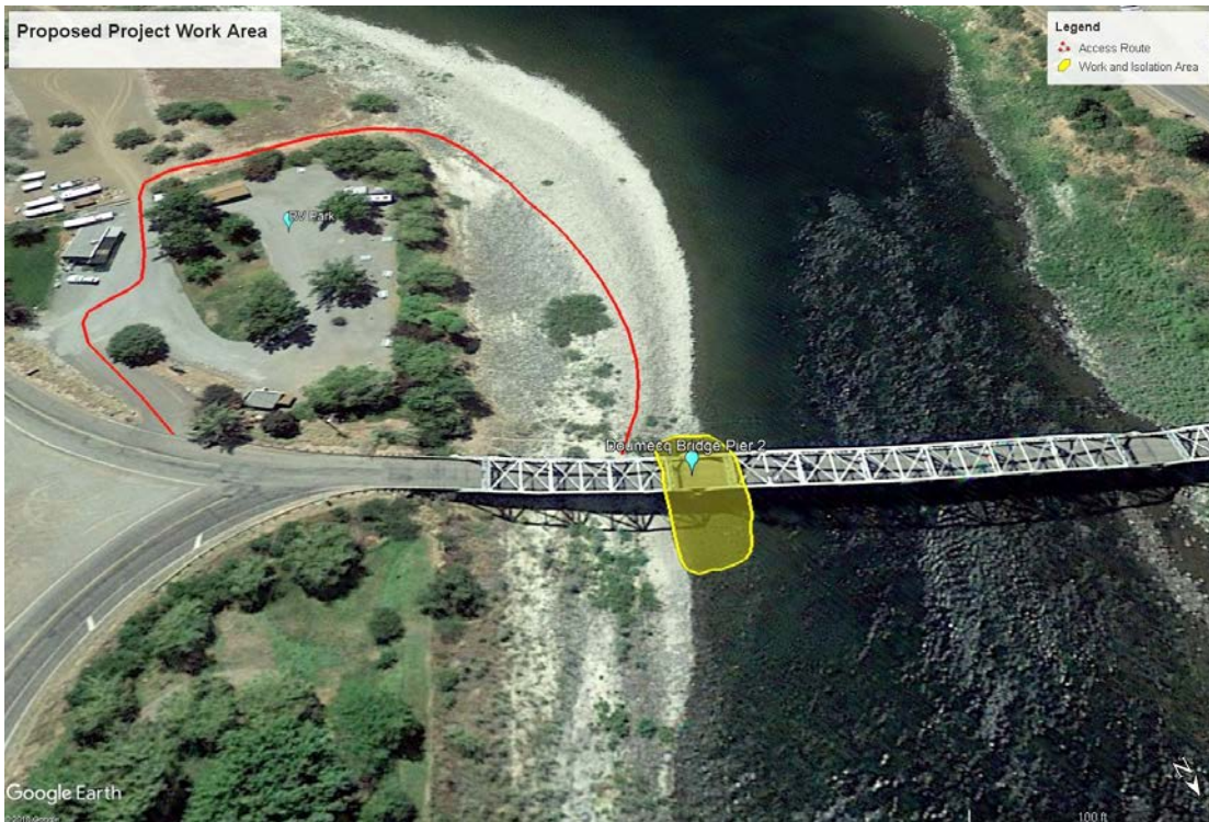
Figure 2. View of Doumecq Bridge work area. The red line indicates the access route for equipment (COE 2019).
