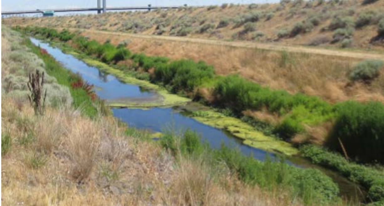
Figure 16. McNary levee system ditch, showing typical vegetation management and exposed water.
