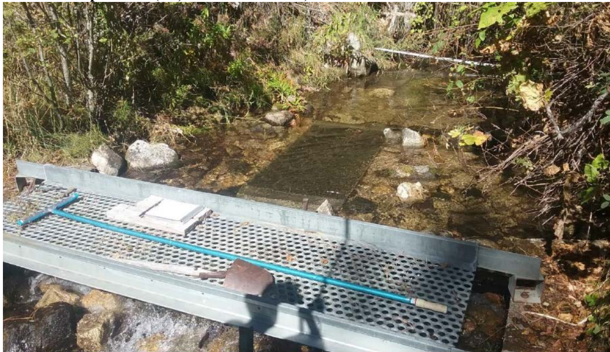
Figure 2. Point of diversion for the Smith Creek Diversion showing the Johnson Bar screen, the permanent walkway used to clean the screen, and screen cleaning implements (i.e., broom and shovel).
