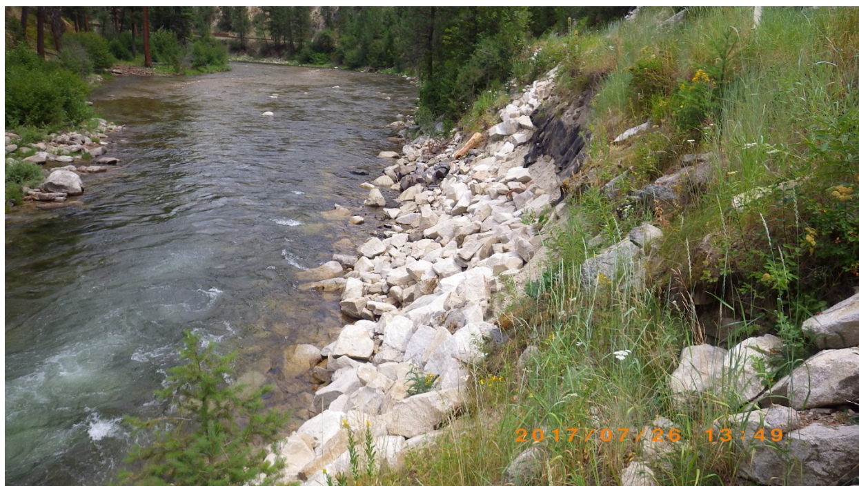
Figure 2. Mile post 23.5 project area showing riprap added by the PNF in 2017, a lack of riparian vegetation along the water’s edge, and an oversteepened condition due to historic erosion.
