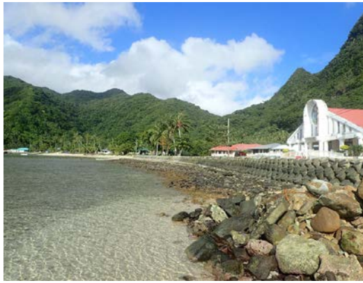
Image 5: Church and surrounding houses in village of Vatia. Seawall is pictured in the foreground.
