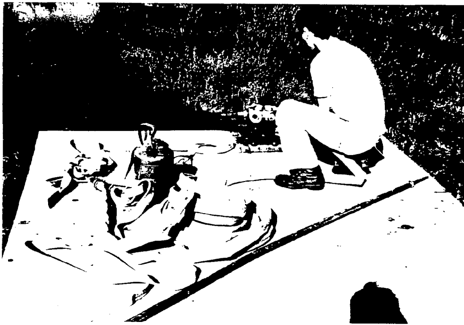
Jetting apparatus, pipe, nozzle, hose and pump.
