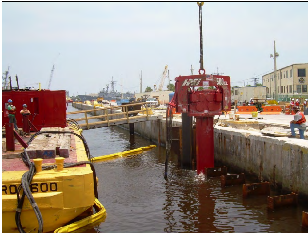
FIGURE 4-2. VIBRATORY INSTALLATION OF SHEET PILES AT NAVSTA MAYPORT
