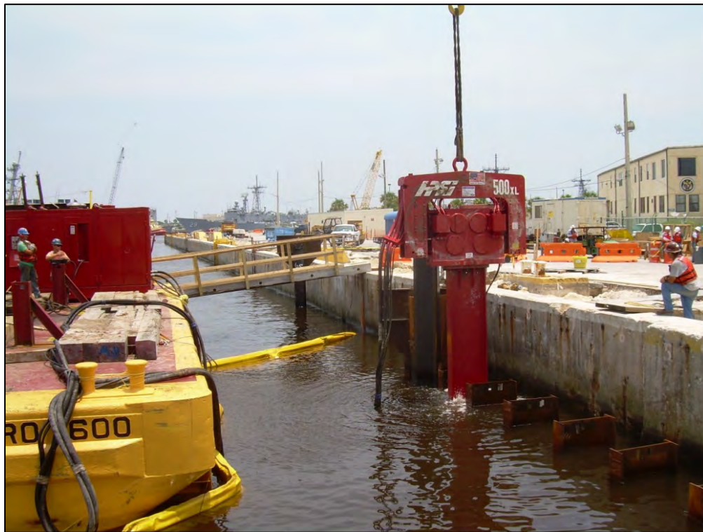
Figure 2-2. Vibratory Installation of Sheet Piles at NAVSTA Mayport
