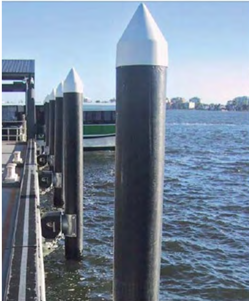
FIGURE 4-4. POLYMERIC FENDER PILES
