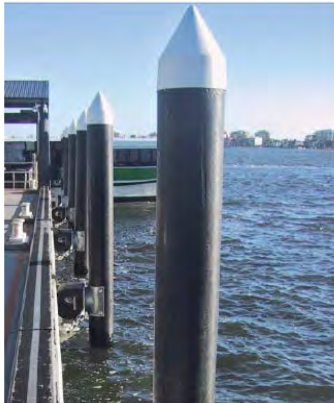
Figure 2-4. Polymeric Fender Piles
