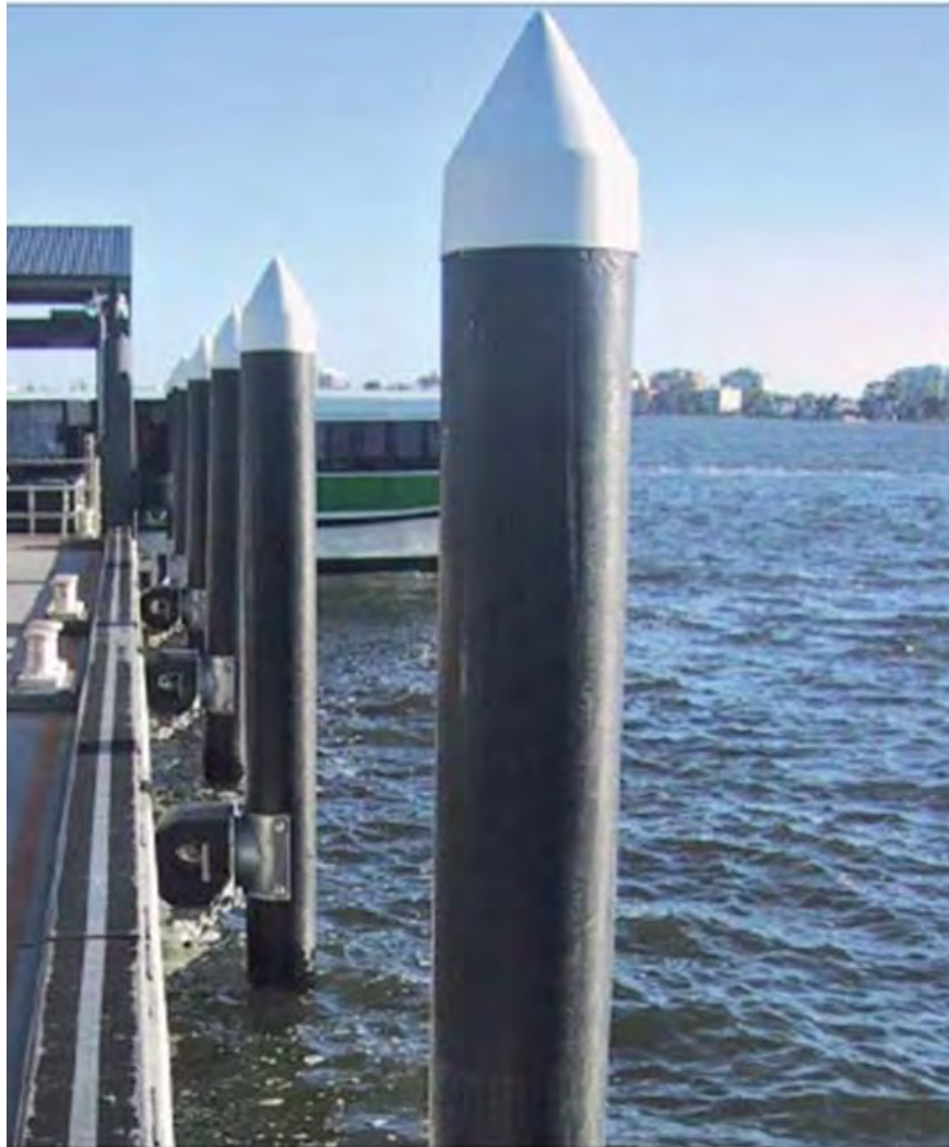
FIGURE 4-4. POLYMERIC FENDER PILES
