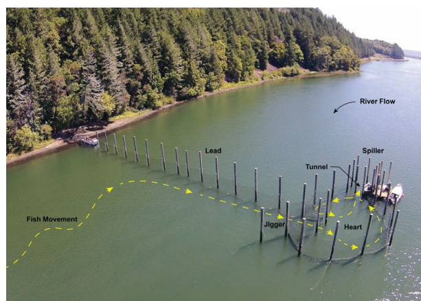
Figure 2. The experimental fish trap in the Columbia River (river kilometer 67) consisted of a lead, jigger, heart, tunnel, and spiller.
