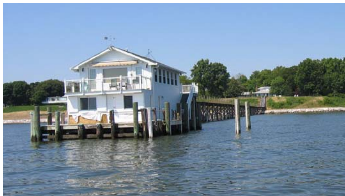
Figure 8. This structure on the Magathy River, Maryland is not water dependent and would not be permitted in Massachusetts.
