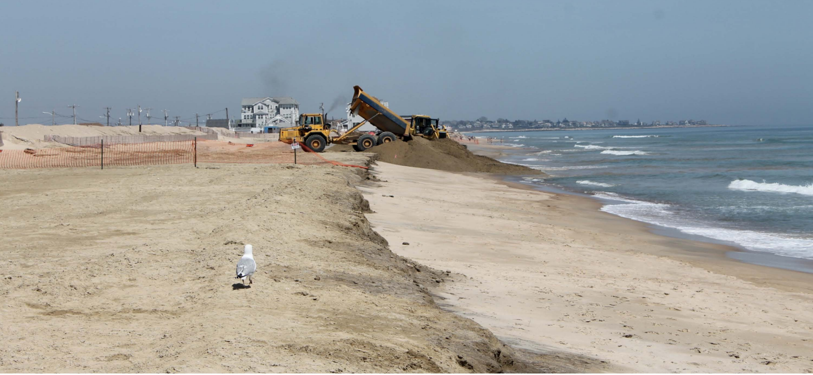
Above, beach restoration efforts. Photo courtesy of Bryan Oakley. At right, Newport Harbor. Photo by Monica Allard Cox.
