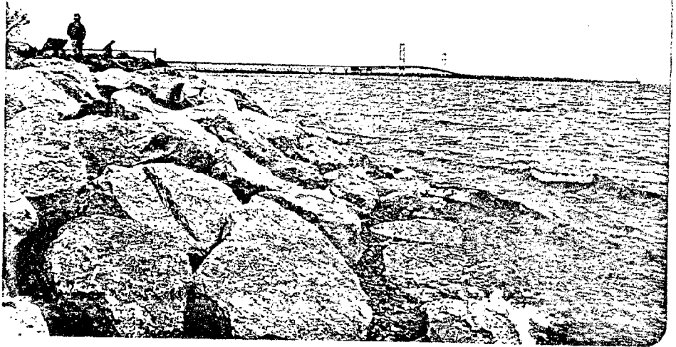
EROSION CONTROL STONE
