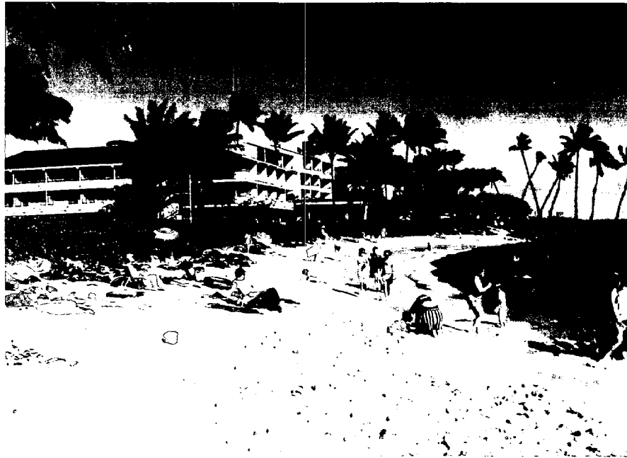
FIGURE 2-5 BURIED REVETMENT AT POIPU, KAUAI
