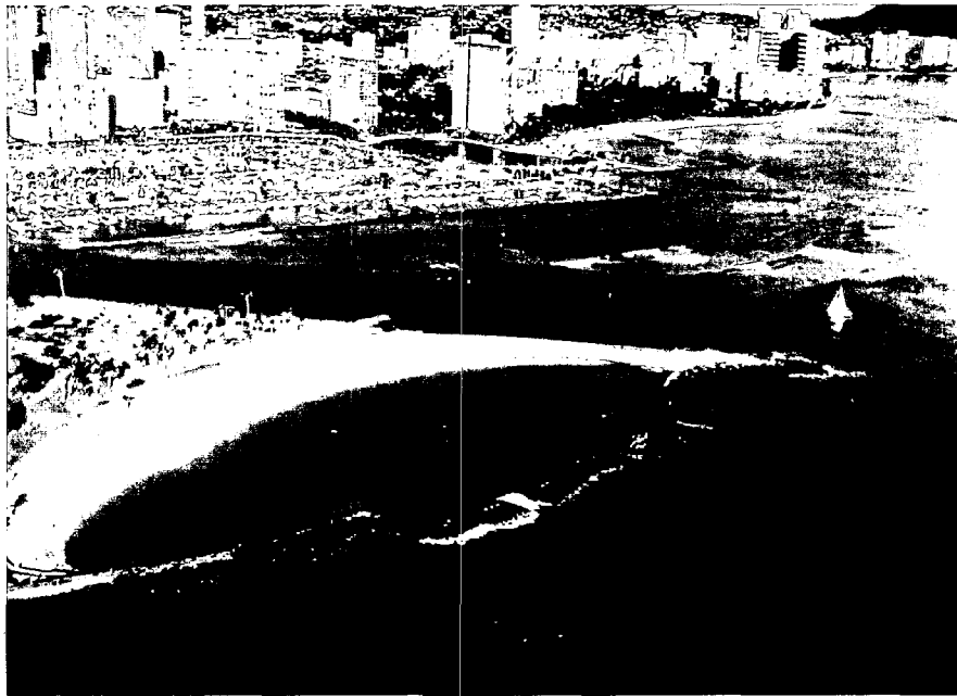
FIGURE 2-9 BEACH FILL WITH CONTAINMENT STRUCTURES AT MAGIC ISLAND PARK, OAHU
