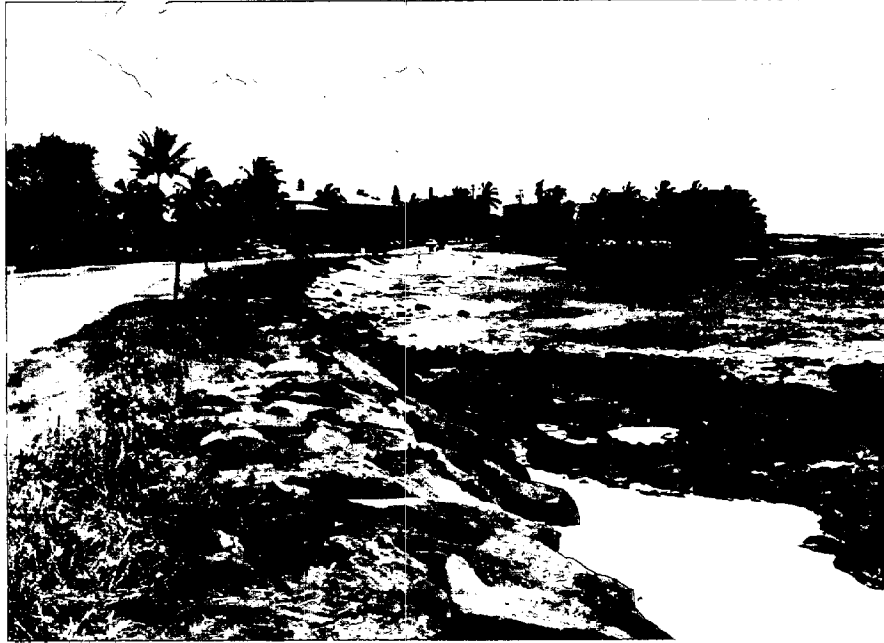
FIGURE 2-4 ROCK REVETMENT AT KUKUIULA, KAUAI
