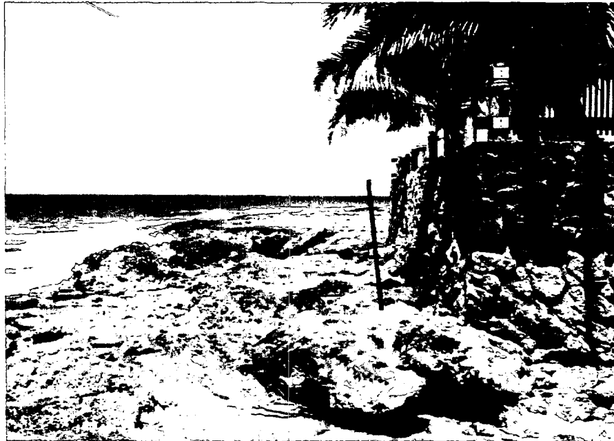
FIGURE 2-3 ROCK MASONRY SEAWALL AT MAKAHA, OAHU
