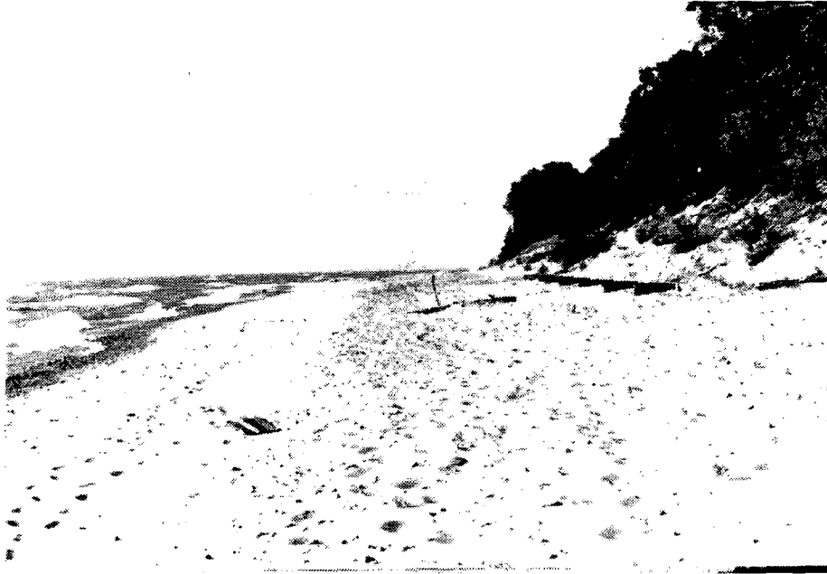
Figure B48. Site S: Looking north at retaining wall just visible at toe of bluff.
