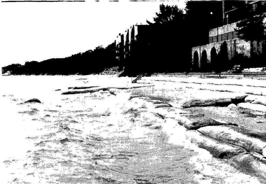
Figure B51. Site U: Looking northeasterly from same point as Fig. B50. Note sand filling behind offshore sill. Beach is beyond sill to the south of this location.
