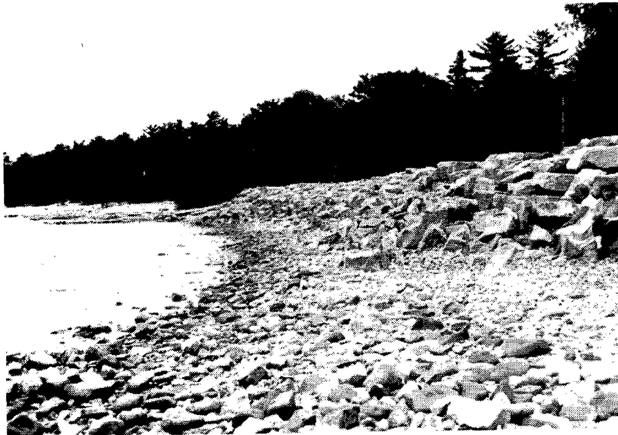
Figure B59. Site W: Looking at coarse beach in front of revetment.
