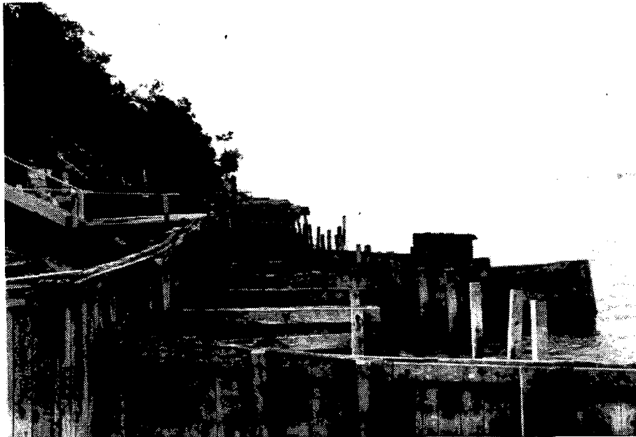
Figure B35. Site L: property just to south of site. Note closely spaced short timber groins projecting from retaining wall.
