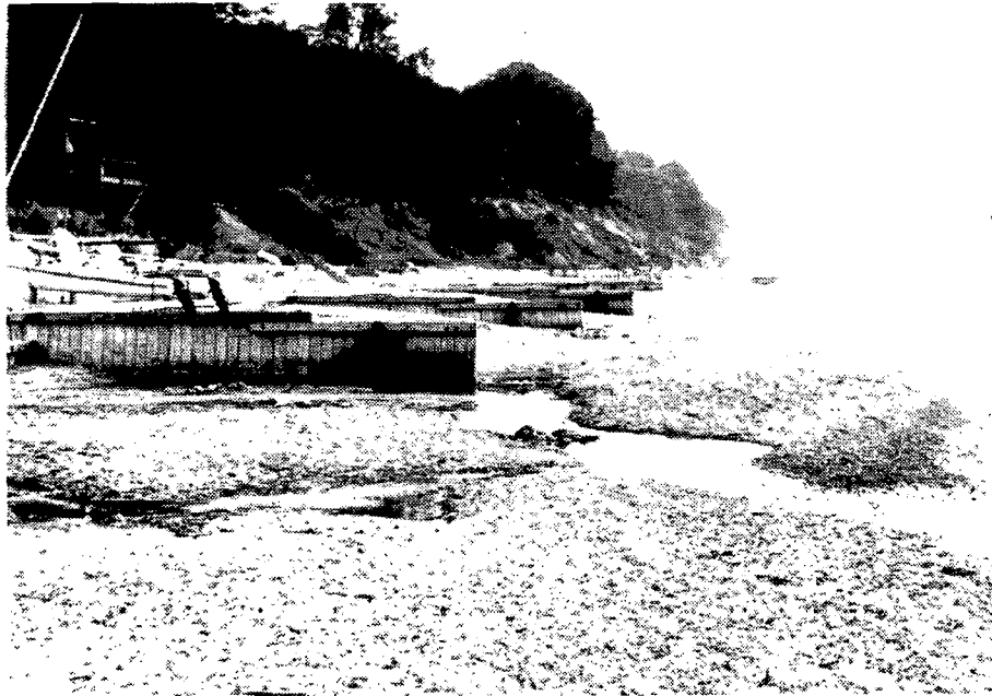
Figure B10. Site D: View of groin system on south side of creek. Decrease in beach width to the south is fairly clear in this photograph.
