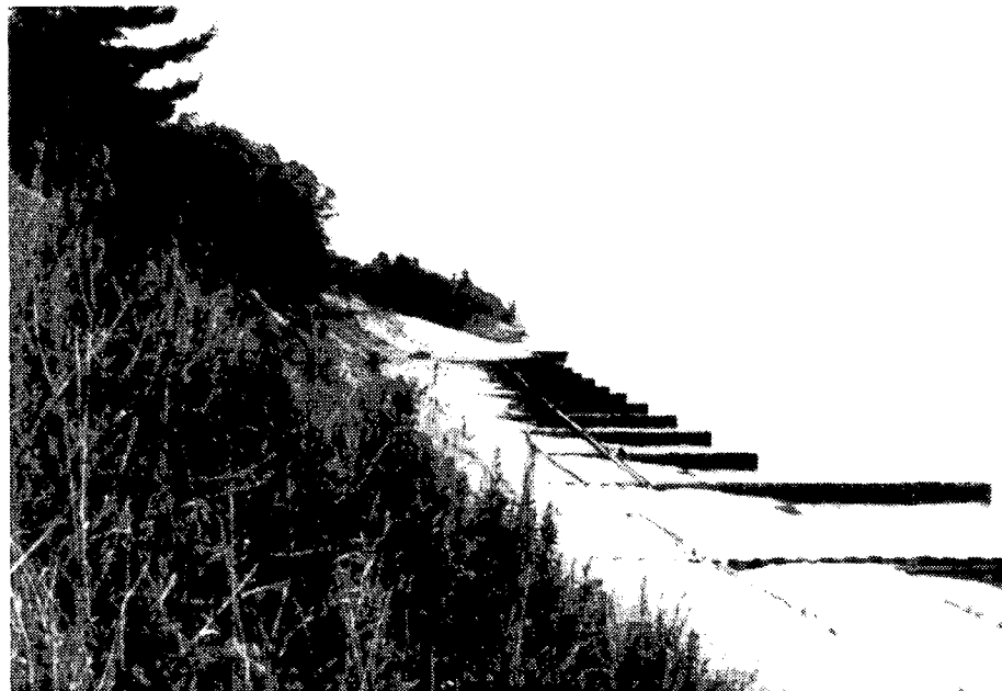
Figure B21. Site H: Looking towards southern end of property from approximately the middle of the groin system. Note that southernmost groins are shorter than the two closest ones. Wavebusters are present in lower right of photo.
