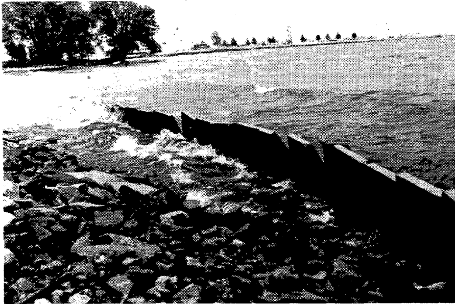
Figure B60. Site X: Normandy type wavebusters in front of 240 S. State. Note revetment almost immediately behind wavebusters.
