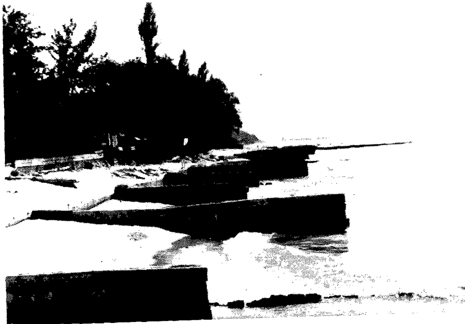
Figure B39. Site M: Looking south from 8th groin north of second long concrete groin.
