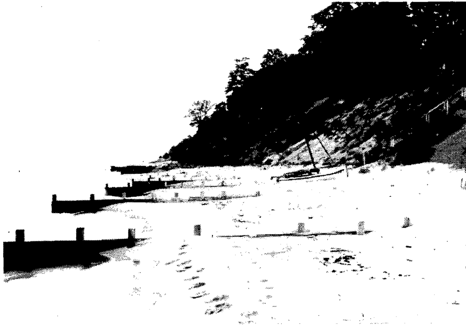
Figure B15. Site F: Looking north towards the site. Buried groin is to the north of the four groins in the foreground. Note longer and higher groins on either side of property.
