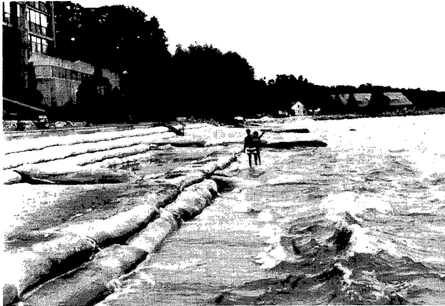
Figure B52. Site U: Looking towards the southwest from the most northerly groin in the system. Beach is higher behind bathers, may be due to artificial filling or littoral drift from the southwest.
