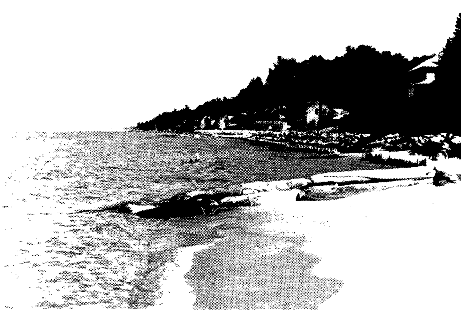
Figure B24. Sites I and J: Tube groin (part of Reid permit) on south boundary of Epworth property. Note accumulation of beach on south side of groin and slight accumulation behind other tube groins to north (in vicinity of old timber retaining wall).
