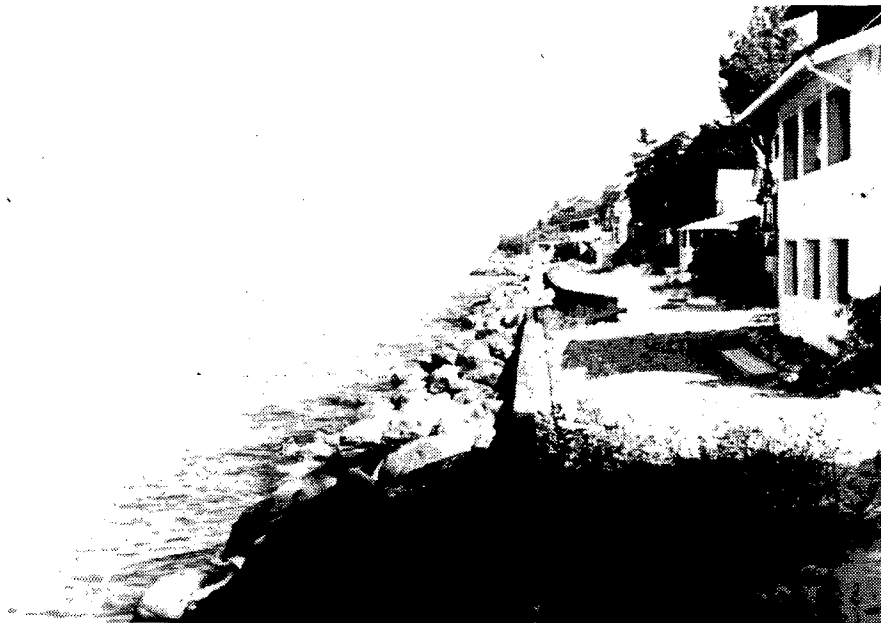
Figure B27. Site J: Closer view of revetment at location where it is backed by a retaining wall.
