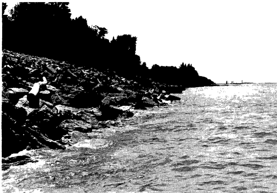
Figure B41. Site O: Looking south along revetment from location in Fig. B36 where abrupt turn in shoreline occurs.
