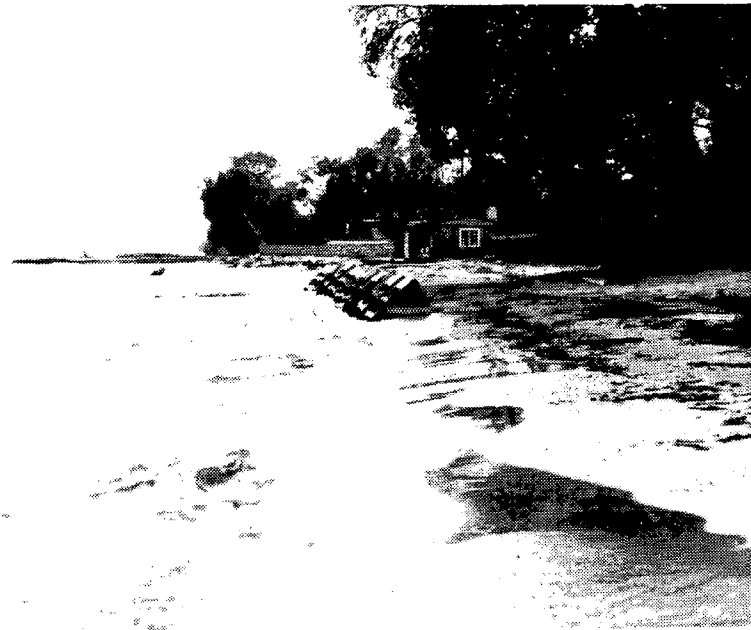
Figure B62. Site X: Looking south at wavebusters at 430 S. State. Note shore protection allows property to south to project farther lakeward.
