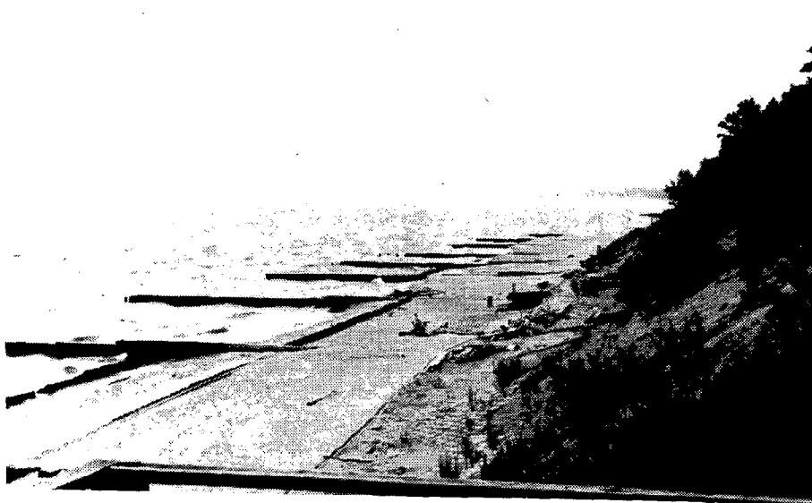
Figure B19. Site H: View towards the north of the last eight groins at the northern side of the system. Tops of wavebusters are visible at lower left side of photograph. Flex-blocks are visible in foreground at toe of bluff.
