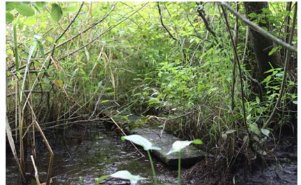
Figure 6. Existing duck hunting catwalk at the site of the preferred alternative.
