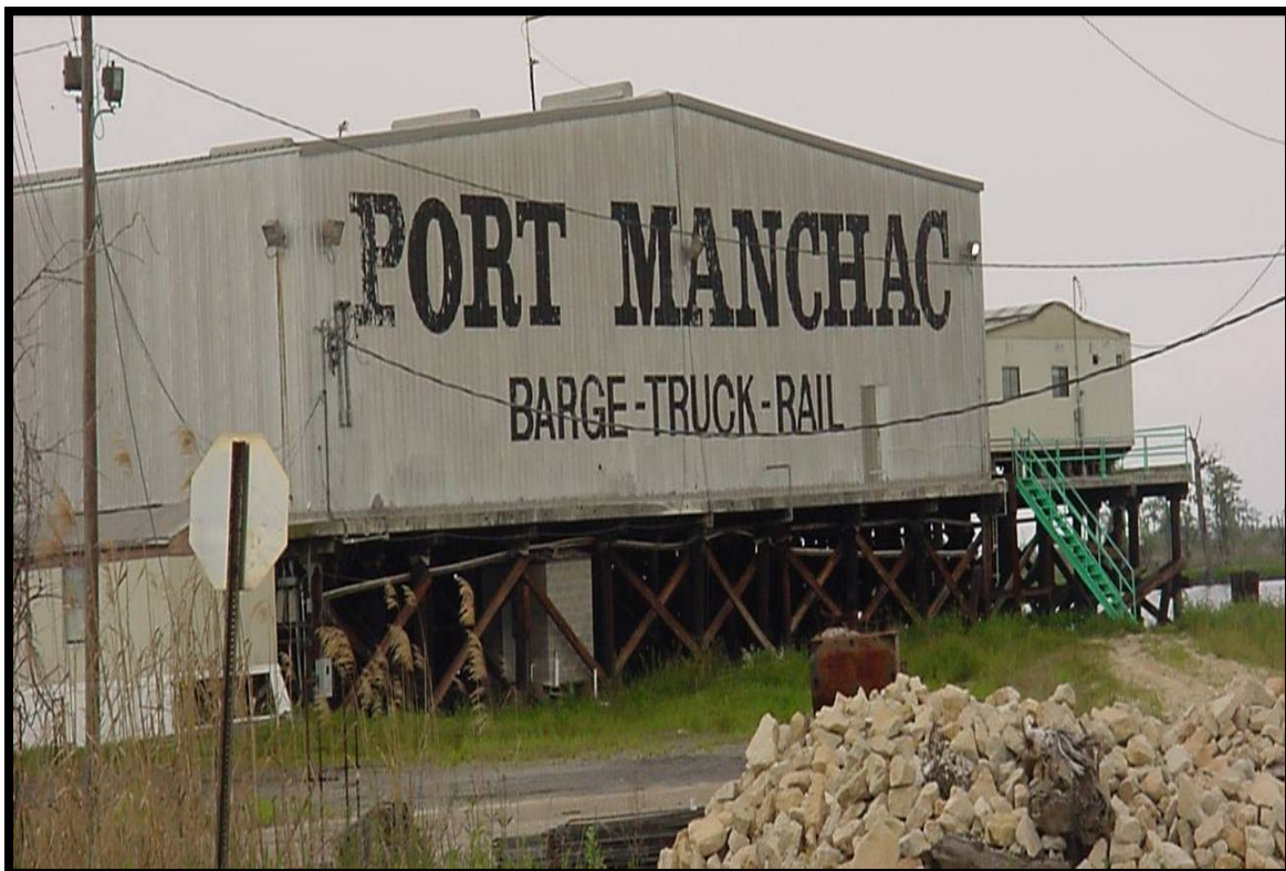
Port Manchac Railroad-Barge Interface Facility
