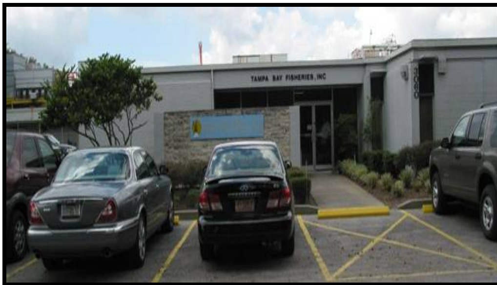
Fish Processing Facility in Dover
