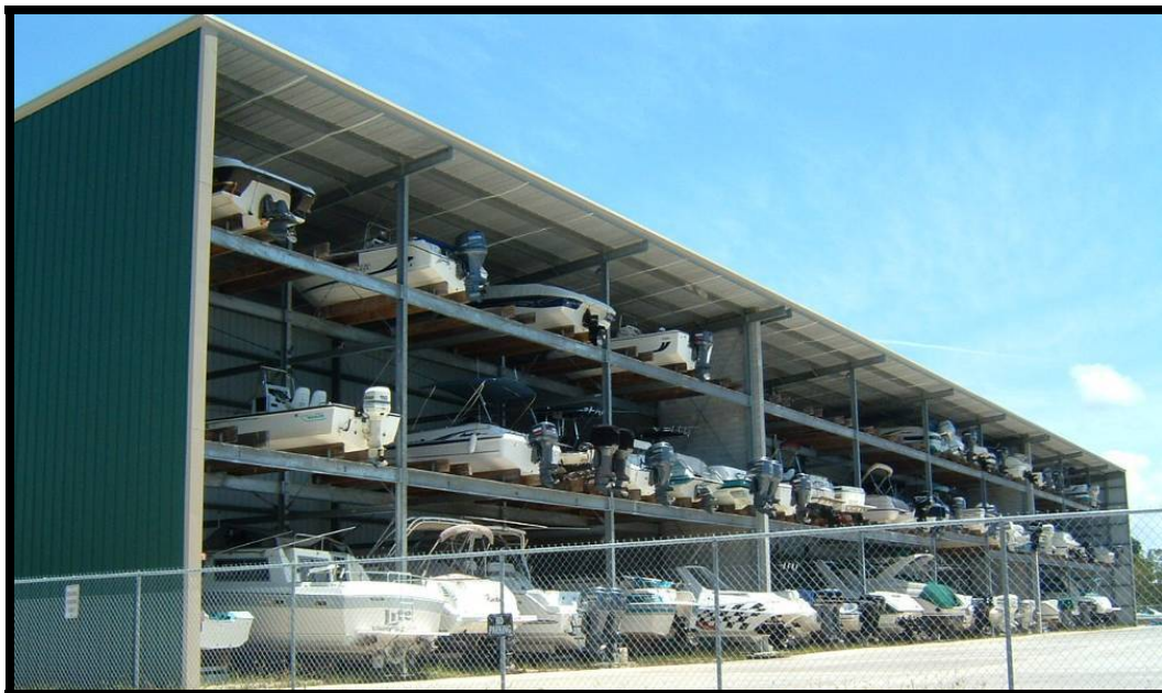
Dry Dock Storage at Goodland Marina
