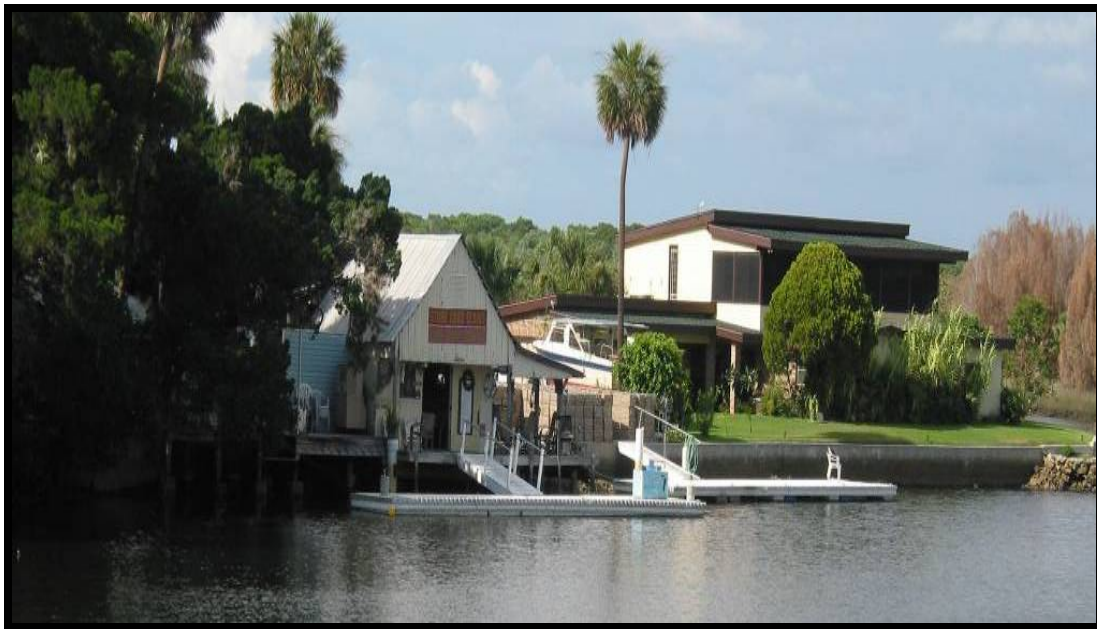
Former fish house in Aripeka
