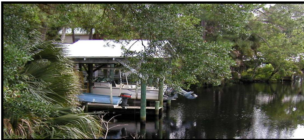
Mooring Canal at Horseshoe Beach
