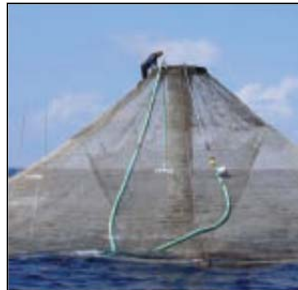
Figure 19 The SeaStation, seen here on the surface, is a type of fully submersible net-pen.
