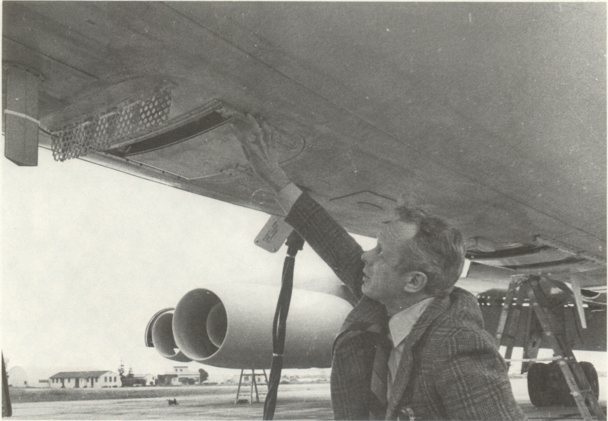
Figure 1. Convair 990 aircraft installation for infrared imager.
