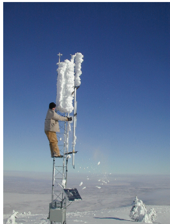
Figure 86. Technician removing rime ice on meteorological tower on the top of Big Southern Butte, in January 2002.
