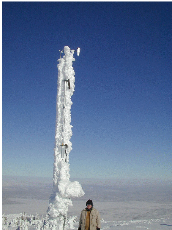
Figure 85. Extreme rime icing on meteorological tower on the top of Big Southern Butte, in January 2002.
