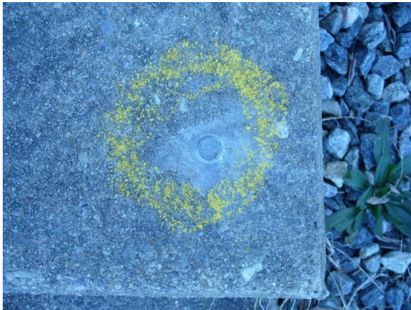
Figure 10 - Permanent Bench Mark (PBM 1) at office steps.
