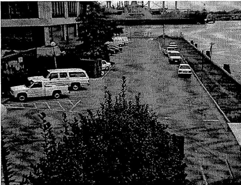
Figure 3-1. Parking lot behind Portsmouth City Hall considered for the Delaware Sand Filter design. The catch basin that serves this lot is located beside the second vehicle on the right side. The filter would be located in the grass area adjacent to the Elizabeth River.
