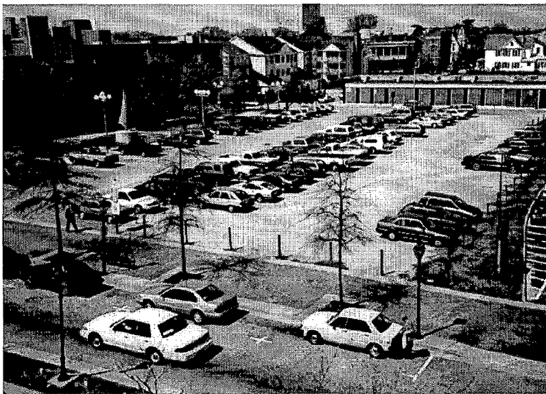
Figure 3-3. Parking lot on High Street considered for the D.C. Sand Filter design. The left half of the parking lot is asphalt with a drop inlet that can be seen just above the center of the photograph. The right half of the lot is gravel with no internal drainage structures.
