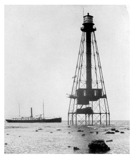
Plate 7. Sombrero Key lighthouse (19--). The lighthouse was built in 1858 and had iron skeleton tower 160' high. The light is 142' above water. [Photoprint, black and white (10 x 8 in). rc05651. Reference Collection, Florida State Photo Archive. <a href="http://fpc.dos.state.fl.us/>.]</a>.
