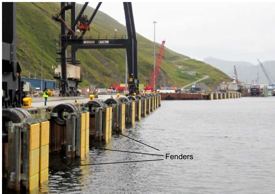
Figure 2. Existing UMC Dock Position V with USCG dock in background. Current project would connect the gap between these with a dock of similar structure.
