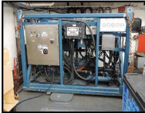
HPU secured to deck using chains
