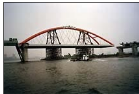
High accuracy height information is critical in bridge construction
