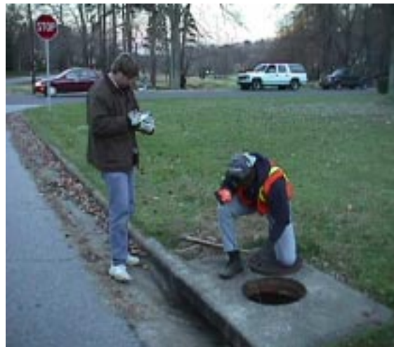
Figure 13 Measuring Invert Offsets for a GPS RTK Survey of Sewer Pipes
