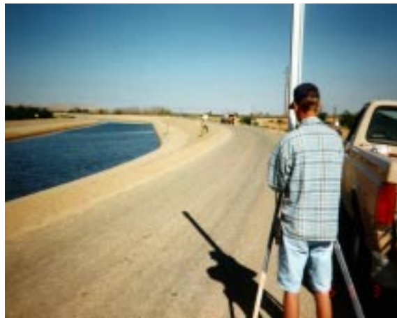
Figure 14 Subsidence Monitoring Along an Irrigation Channel
